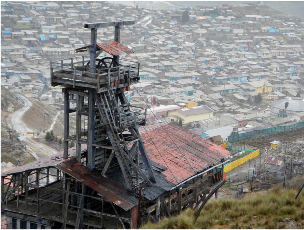
Figure 2. The Elvira Headframe, overlooking the town of Quiruvilca. R. McDougall photo.
