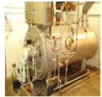
The following is an analysis of the gas usage since installation of PC Fuel Optimizer on a single boiler at one High School with two further sets of adjustments to try optimize the set up. The boiler was a Black & McDonald Combustion set up and the engineer in was T. Wiggins. The boiler test was on a Power Master boiler, model 3LG Serial Number 695\*\*\*3, 500 HP, 60 PSI, Natural Gas, 20,900 cu. Ft/hr.
