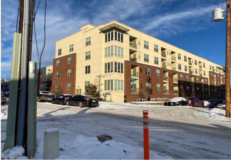
View of northwesterly adjoining 2785 Speer mixed-use retail/residential building. View to the northwest.
