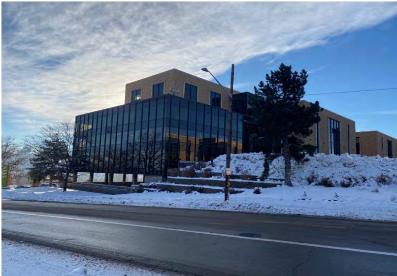
View of southerly adjoining Diamond Hill office building. View to the southeast.
