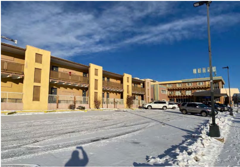
View of typical site conditions. View to the north.
