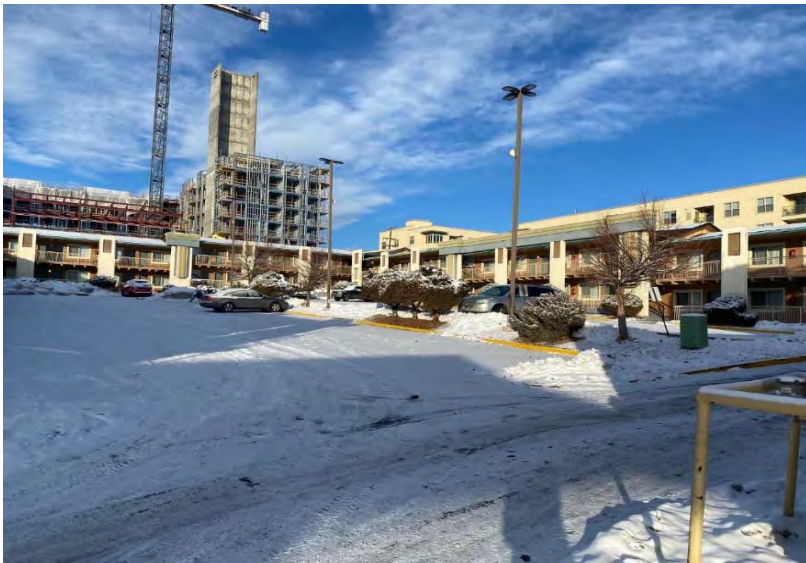
View of typical site conditions. View to the northwest.
