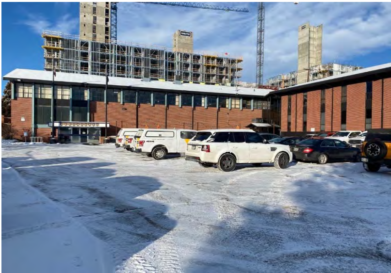
View of southwesterly adjoining Elks Lodge 17. View to the west.
