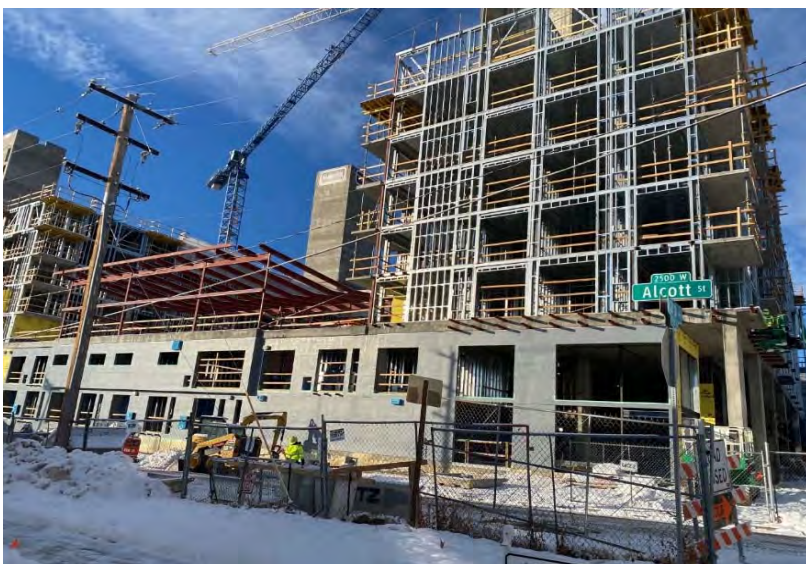
View of westerly adjoining land under construction. View to the southwest.
