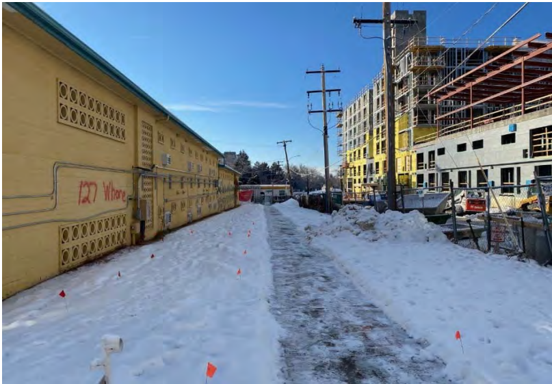
View of typical site conditions. View to the south.
