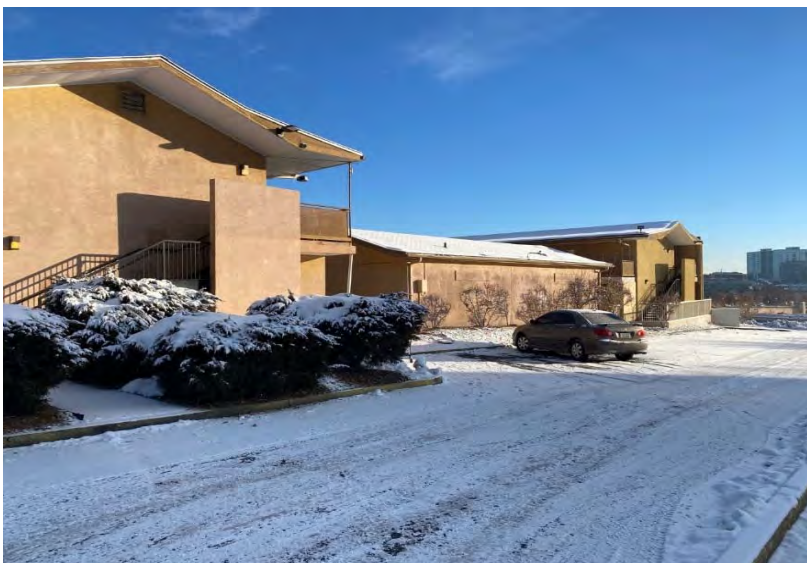
View of typical site conditions. View to the northeast.
