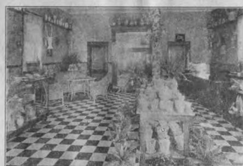
An Interior View of the Woodbridge Flower Shoppe which measures 28ft.x40ft. and is completely equipped with modern improvements. The walls are stippled paint finish above and colored tile below.
