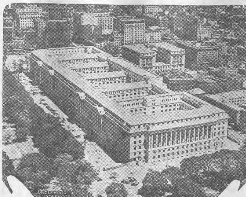
Complete and almost ready for occupancy, the mammoth new home of the Department of Commerce looms prominently in the sky line of downtown Washington. Extending for a distance of three city blocks north and south and a block wide, it is the largest federal office building in the United States.
