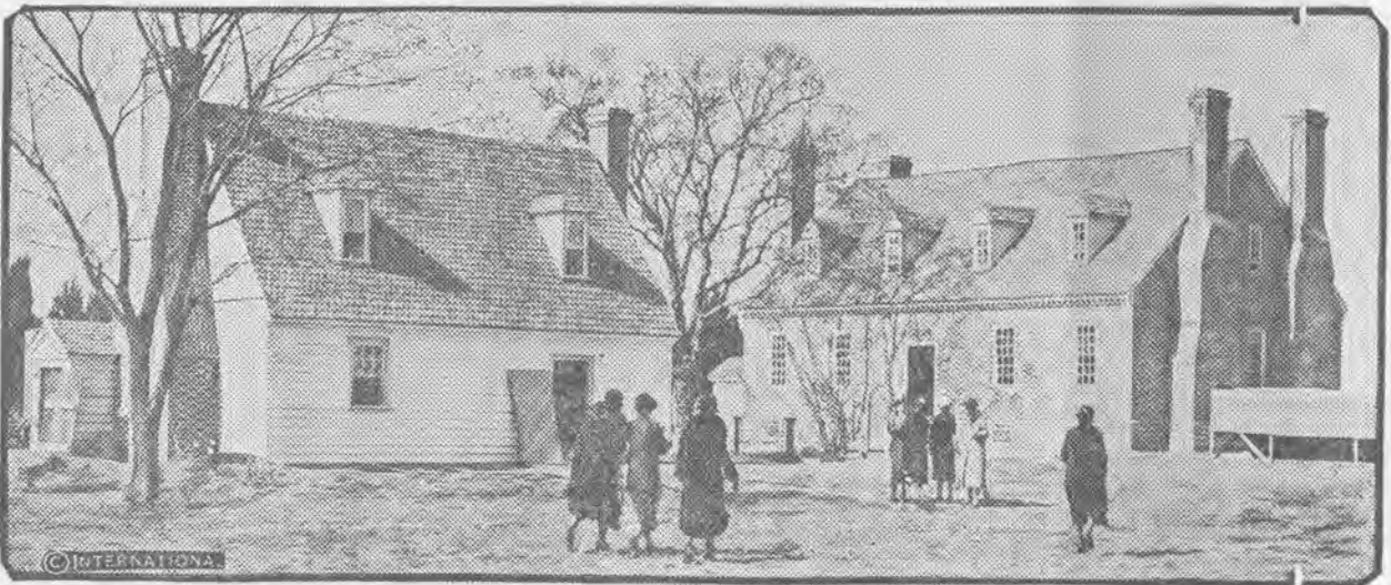
Kitchen and main house of the restored birthplace of George Washington, which is rising from the fire ruins of 150 years ago. The beautiful estate in Westmoreland county, Virginia, is being reconstructed by the government to form an almost perfect reproduction of the house and grounds as they were during the youth of the first President. The work will be completed in time for the George Washington bicentennial in 1932.
