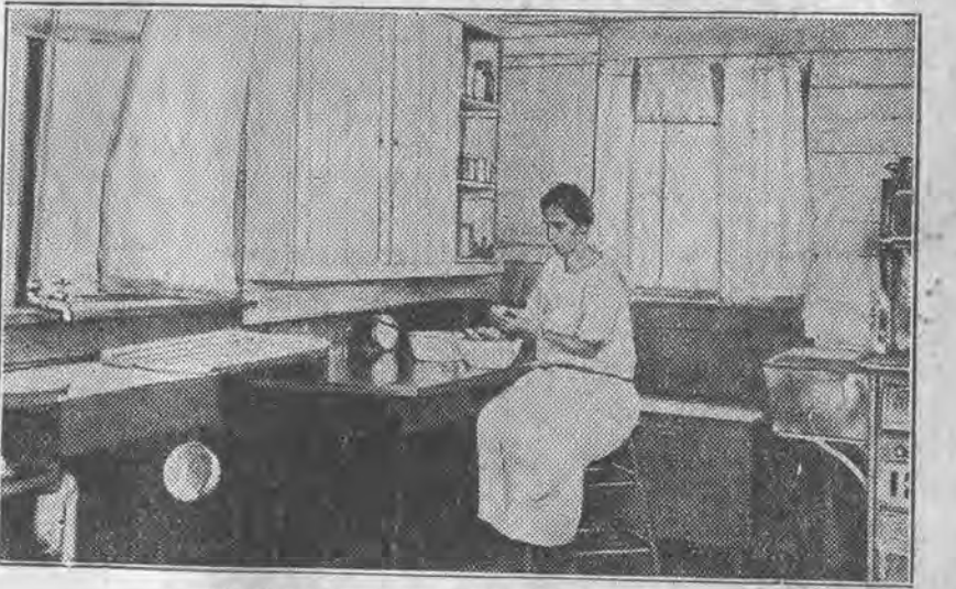
Work Centers Well Placed in Farm Kitchen.
