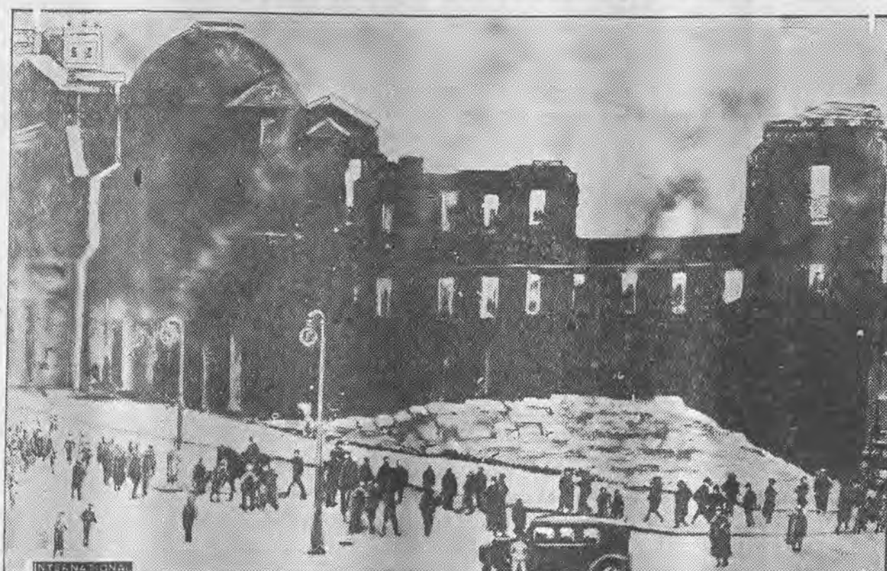
This picture, transmitted by radio and telephoto, shows the ruins of a big Jesuit church in Madrid, Spain, after it had been burned by the anti-clerical rioters.
