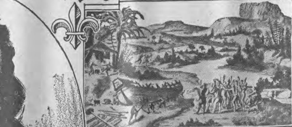
Building of the Griffin
