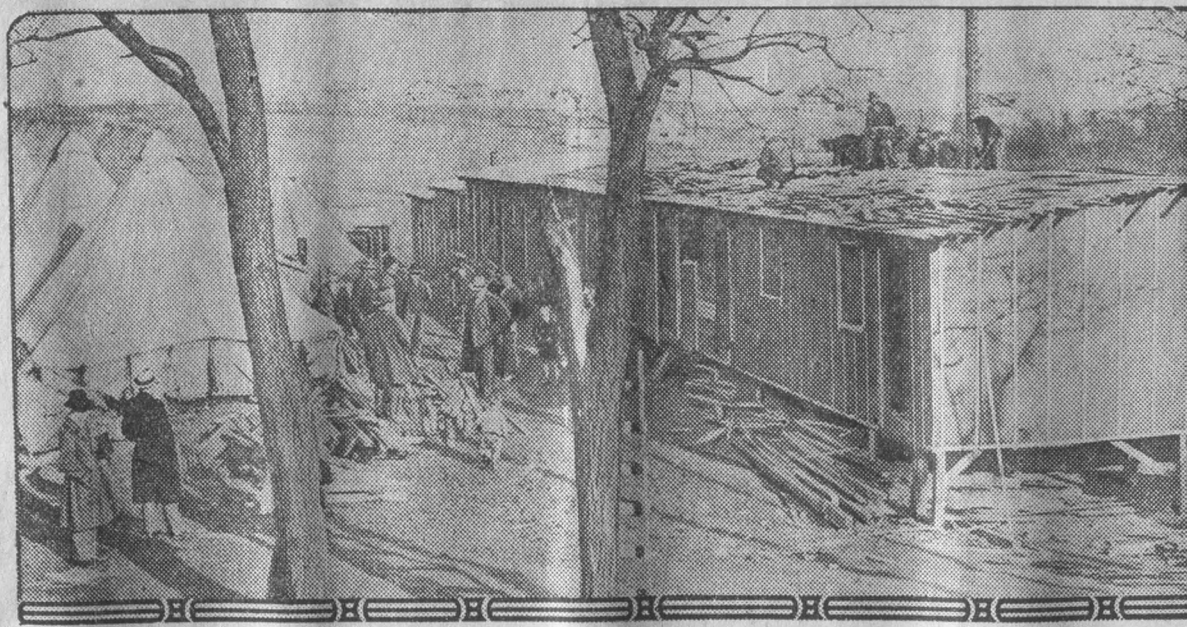
This photograph shows one of the new barracks, each having two rooms, that have just been erected for the evicted striking miners of Coverdale, Pa., by L. G. Altmyer, a Pittsburgh produce broker. At the left are some of the tents that sheltered the miners and their families before the barracks were erected.
