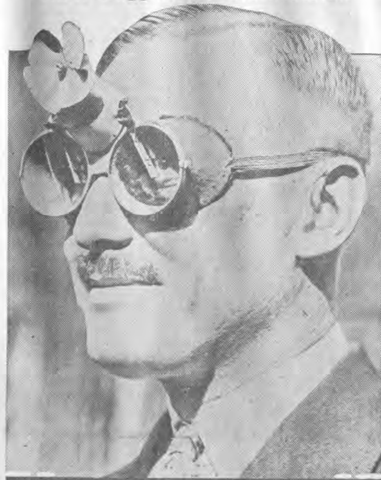
This is L. A. V. Davoren of England wearing a pair of the "rain goggles" that he has invented. They are fitted with windscreen wipers which are driven by an exterior air fan that comes into operation when the motorist is traveling at a speed of fifteen miles an hour or upwards.
