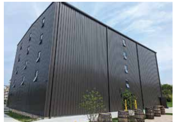
The exterior of the warehouse, the only one of its kind in Pennsylvania, built by experts from Kentucky
