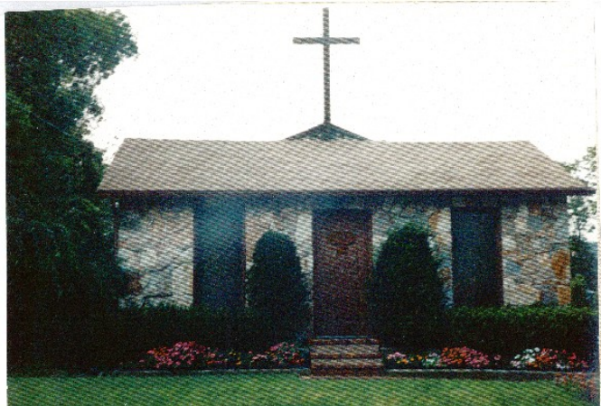
Raintree Irrigation ...Office and Staff meetings held here
