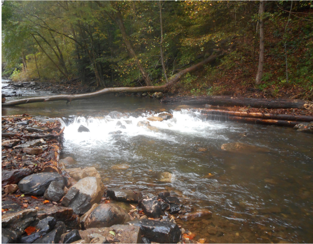
Newly constructed crossvane on Dunbar Creek
