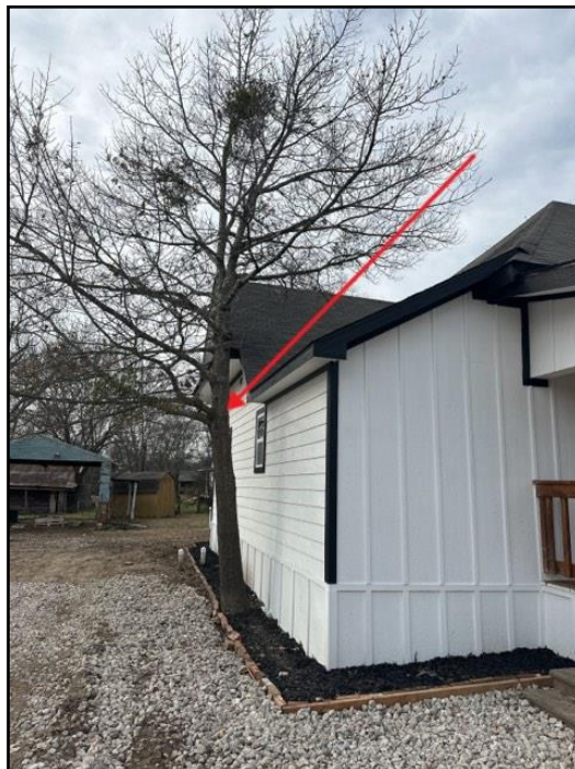
22. Large trees close to building
