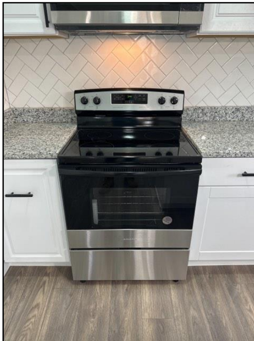
69. Anti-tipping device missing
