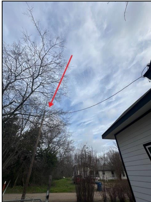
27. Branches / vines interfering with wires
