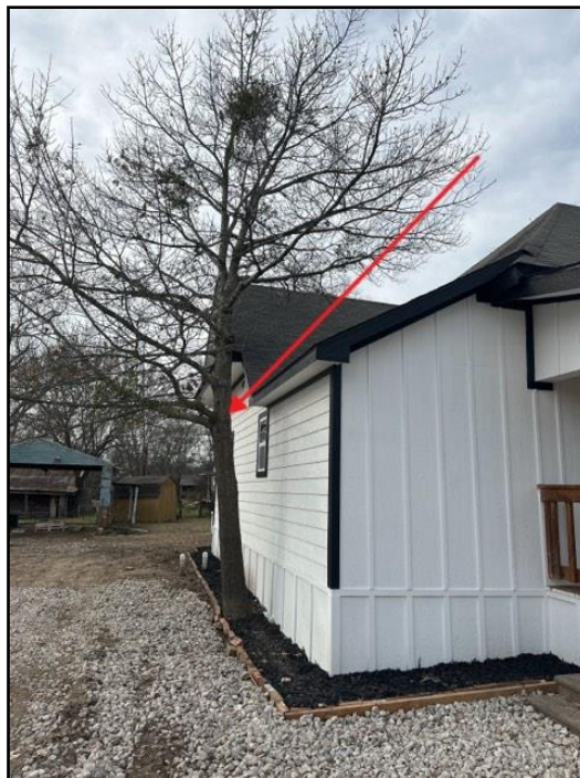
31. Large trees close to building
