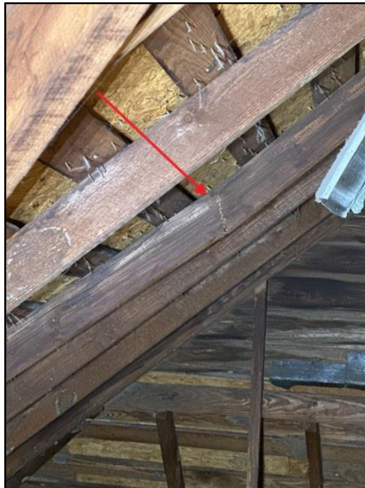
34. Rot, fire or insect damage
