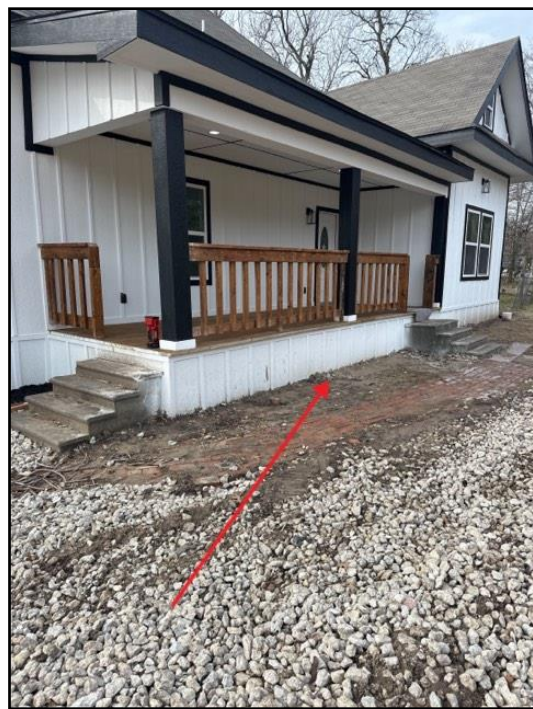
24. Wood/soil contact
