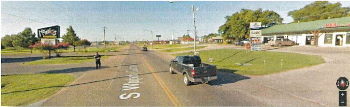
Sidewalks lack connectivity along a commercial strip on State Highway 27, Okemah
