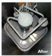
After a thorough cleaning of all components from dirt and mineral oils, the entire refrigeration system is sprayed with SaltShield™ using a custom spray gun for optimal coverage.
