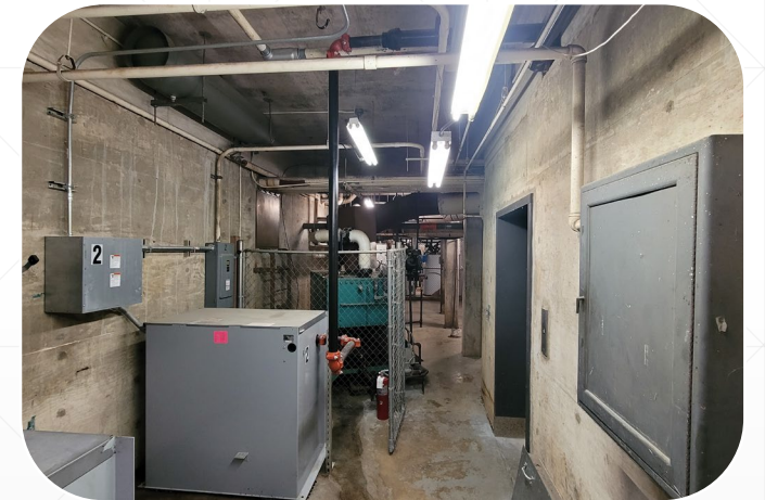
Fence Guard at Elevator
