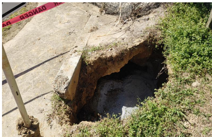
Looking down the hole
