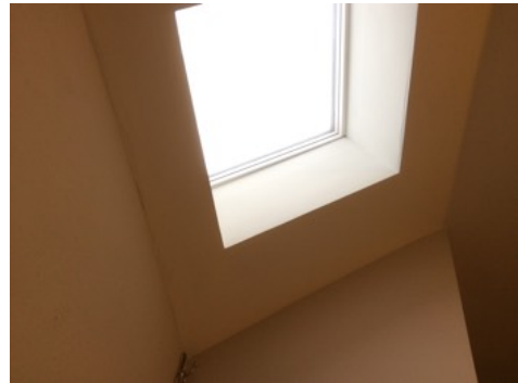
Interior of skylight, no staining
