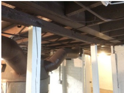
Bracing added to try to relevel floor
