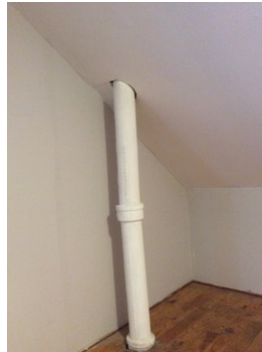
Waste vent pipe - no visible stains
