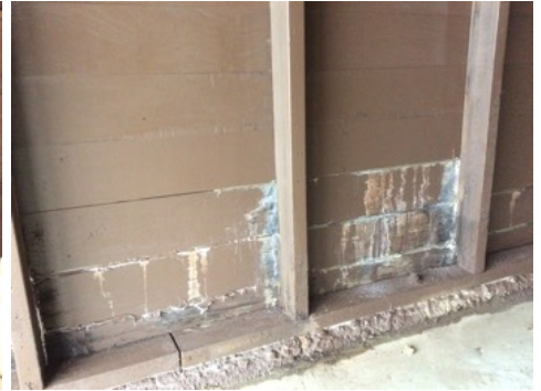
Water staining on recently painted walls
