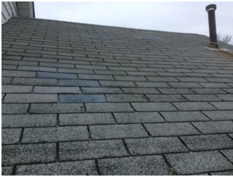
Repair work noted
