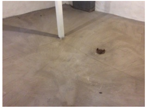
This floor drain was not evaluated
