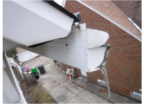
Seal gutter seams
