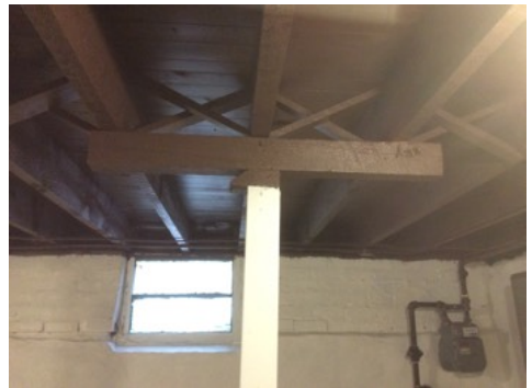
Additional bracing added
