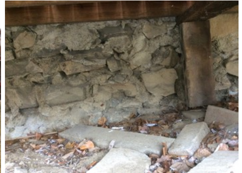
Stone walls - view under porch
