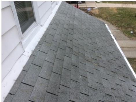
front porch roof
