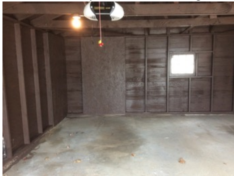
Walls have boards covering sections
