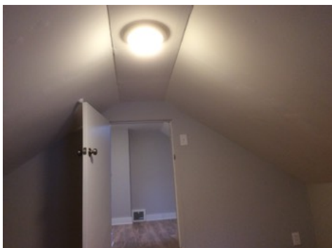
No visible upper attic
