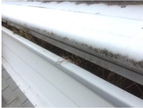
Clean out debris
