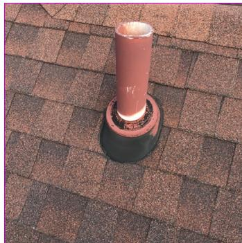
Some flashings were incorrectly installed & do not fully serve their intended purpose.
