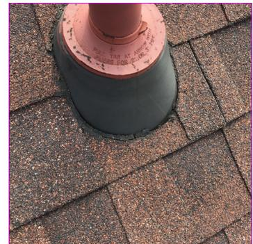
One or more flashing were not properly sealed at the time of inspection
