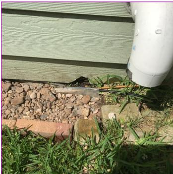
*Sections of the hardboard siding were damaged*
