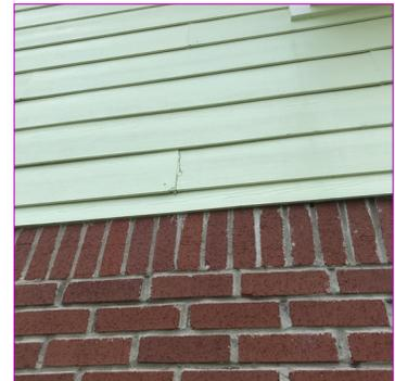
*There were unsealed joints in the hardboard siding. We recommend the joints be caulked or sealed. This is a part of routine homeowner maintenance. Monitor yearly*
