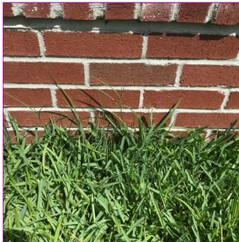
*Foliage is in contact with masonry walls*
