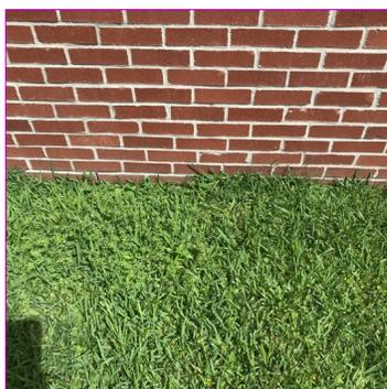
*Soil height close to the exterior facade on part of the structure. This is a path for insects & moisture to travel to enter the home.*
