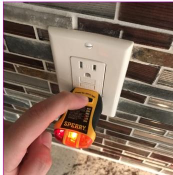
Though the kitchen was equipped with GFCI style receptacles, when tested some of the receptacles did not trip, and therefore, lack GFCI protection
