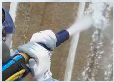
Concrete Surface Preparation
