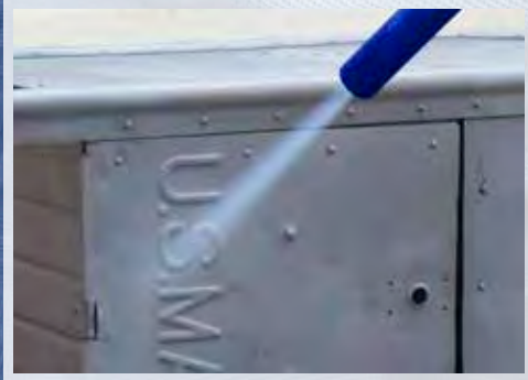
Steel Surface Preparation
