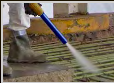
Concrete Repair & Restoration
