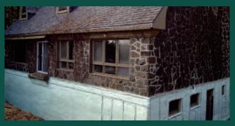
The best way to insulate and waterproof the foundation while keeping cost low, is from the exterior while excavating an existing foundation or before backfilling a new foundation.
