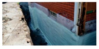
When an old foundation is excavated, it is the ideal time to insulate them by the exterior with spray polyurethane foam.
