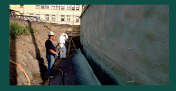
The photo on the left shows a bituminous coating applied directly over spray polyurethane foam. The photo on the right shows a drainage membrane that will be lifted in front of the spray polyurethane foam as the soil is backfilled.
