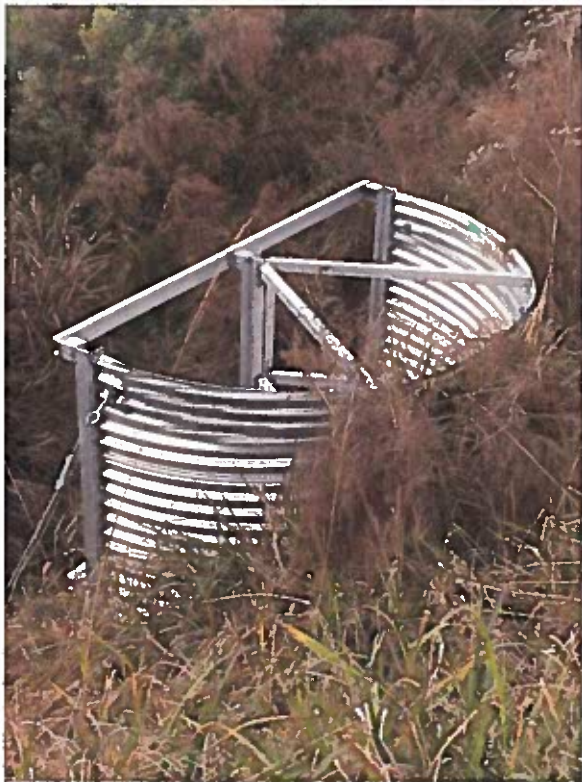
Disposal Area Outlet Structure
