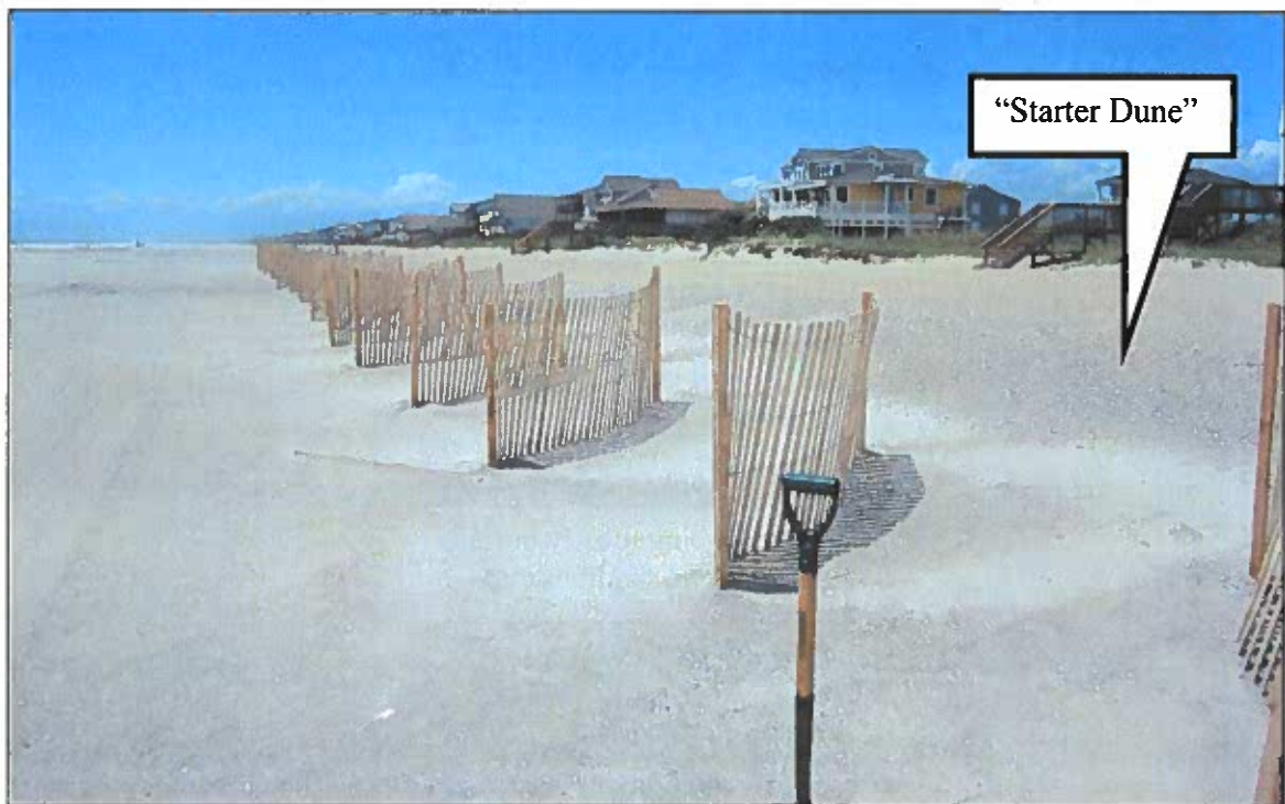
Figure 2-24 (B). Sand Fencing along the Seaward Edge of the Starter Dune for the Central Reach Project at Station ~230+00. Vegetation has been planted on the starter dune since photograph date. (ATM photo, taken May 2017).
