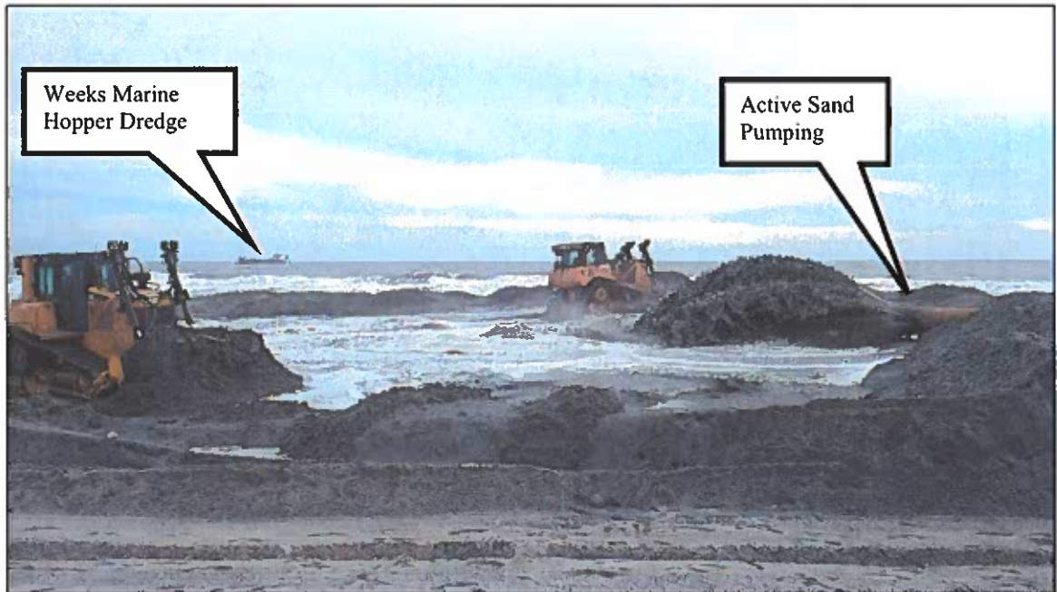
Figure 2-8. Central Reach Construction (ATM photo taken 1/26/17).
