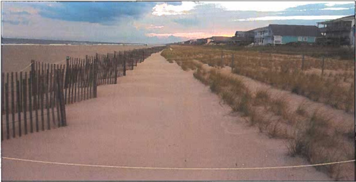
Figure 2-10 (B). Central Reach Post-Construction Approximately Station 230+00 (ATM photo taken August 2018). Note sand fencing, starter dune, and plantings.
