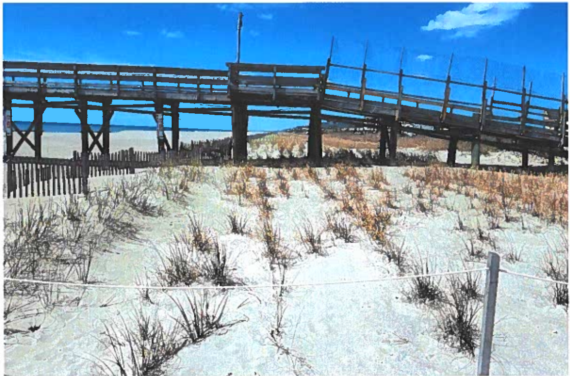
Figure 2-10 (C). Central Reach Post-Construction Approximately Station 170+00 (ATM photo taken March 2019).
