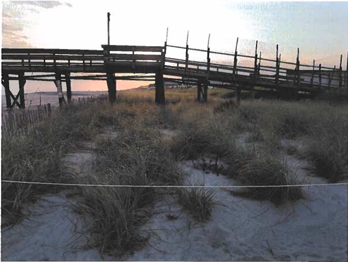
Figure 2-10 (D). Central Reach Post-Construction Approximately Station 170+00 (ATM photo taken September 2019). Note plantings have matured and grown.
