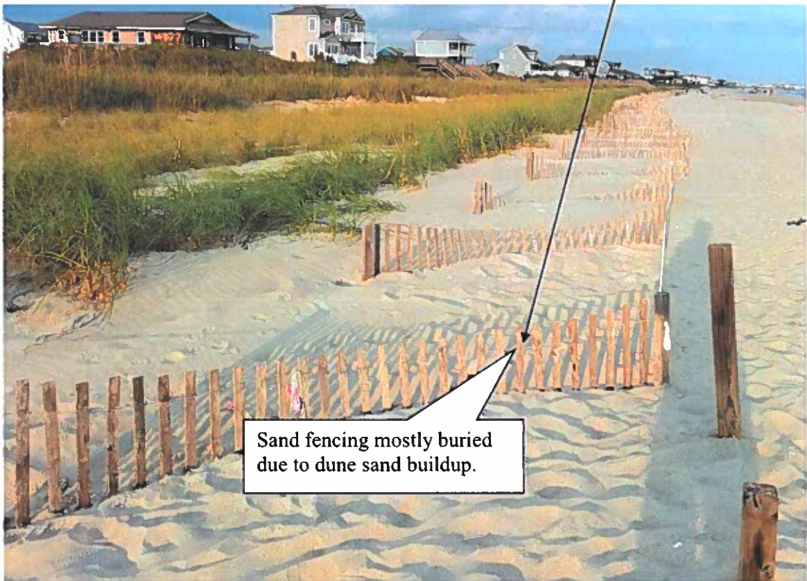
Figure 2-25 (B). Sand Fencing for the Central Reach Project at Station 60+00 showing dune vegetation and sand growth about 2-years post project. (ATM photo, taken September 2019).
