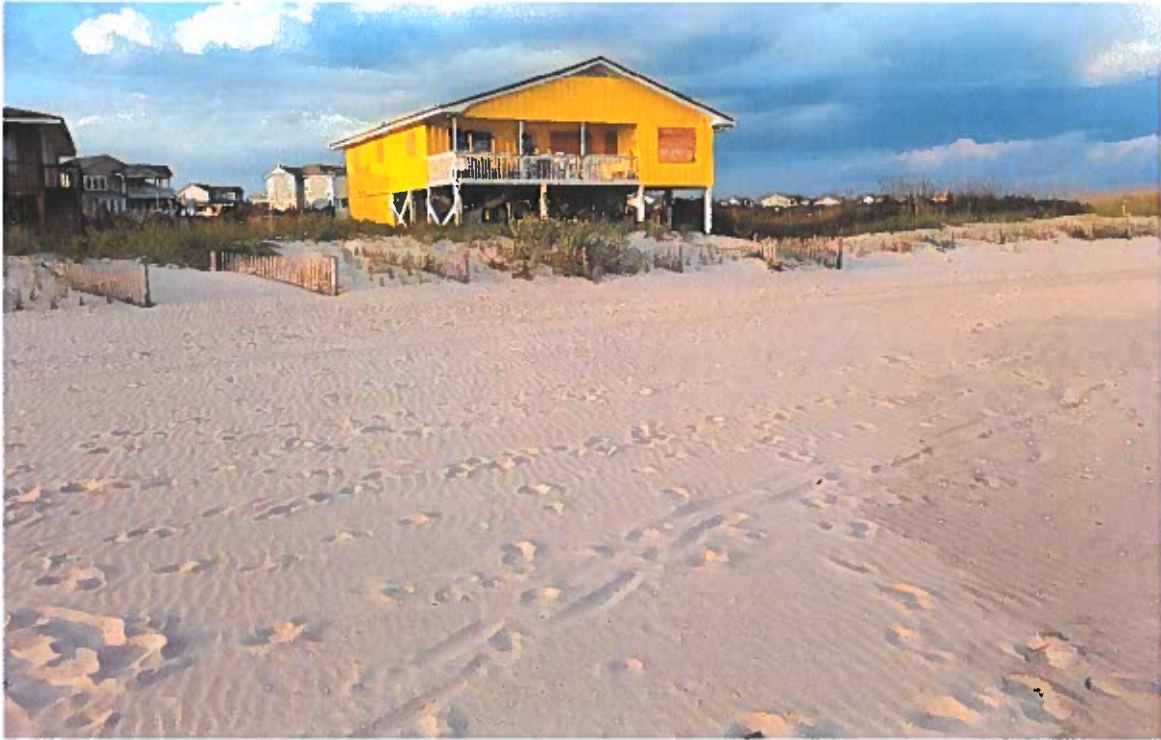
Figure 2-17. Two-Year Post Construction Photo of the 2017 Eastern Reach Project (ATM photo taken April 2018, at Station 20+00). The most eastern oceanfront house, Amazing Grace, is shown. Dune growth has occurred however this is still a vulnerable area.
