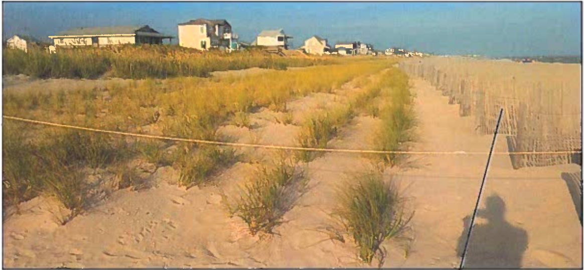
Figure 2-25 (A). Sand Fencing along the Seaward Edge of the Starter Dune for the Central Reach Project at Station ~60+00 Showing Planted Dune Vegetation. (ATM photo, taken August 2018).
