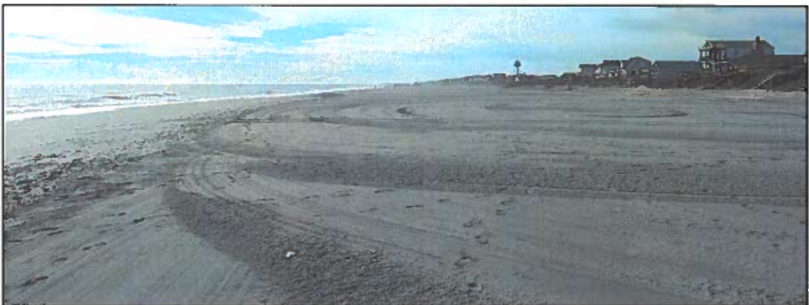
Figure 2-11 (A). Central Reach Immediate Post-Construction Approximately Station 50+00 (ATM photo taken January 2017)
