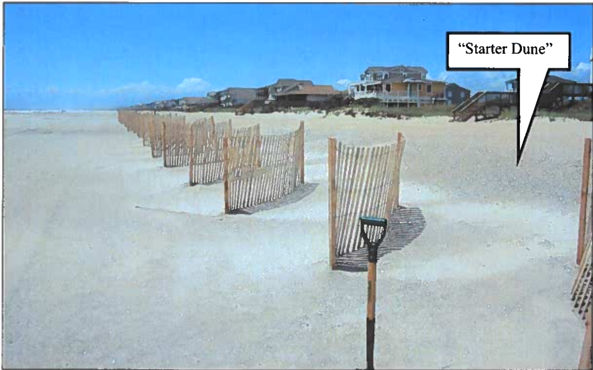
Figure 2-29 (B). Sand Fencing along the Seaward Edge of the Starter Dune for the Central Reach Project at Station ~230+00. Vegetation has been planted on the starter dune since photograph date. (ATM photo, taken May 2017).
