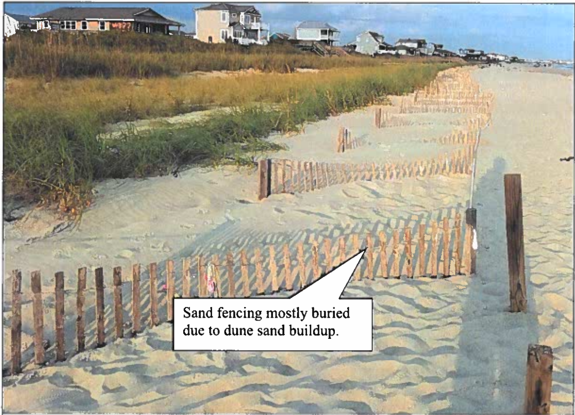
Figure 2-28 (B). Sand Fencing for the Central Reach Project at Station 60+00 showing dune vegetation and sand growth about 2-years post project. (ATM photo, taken September 2019).
