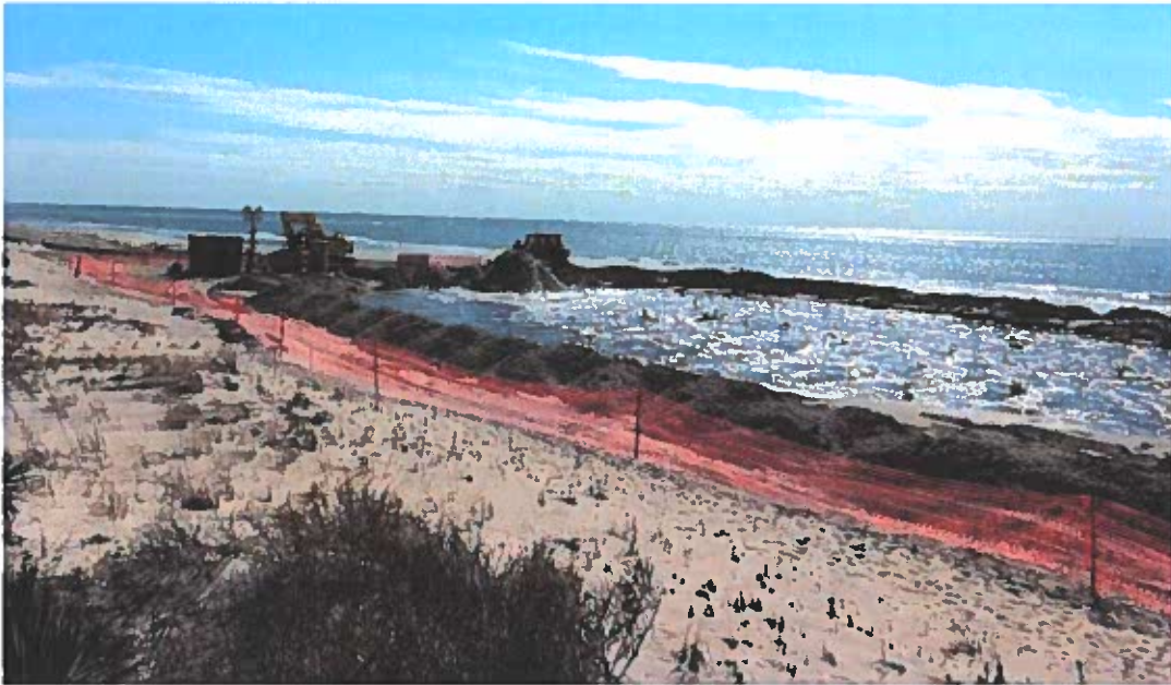
Figure 2-18. Holden Beach POA Photograph Taken near 323 McCray Street (approximately Station 26+00) during 2017 Eastern Reach Project construction.
