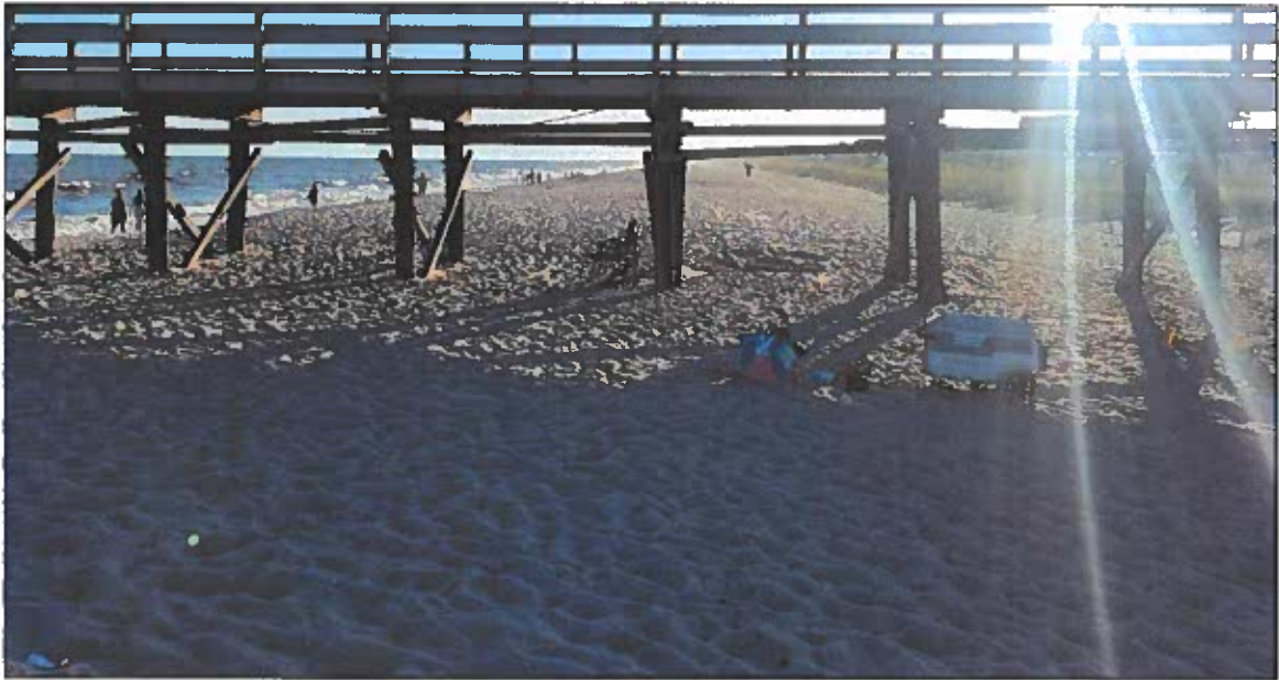
Figure 2-10 (B). July 2020 Photograph Taken Near Pier (~Station 170+00) Looking West.
