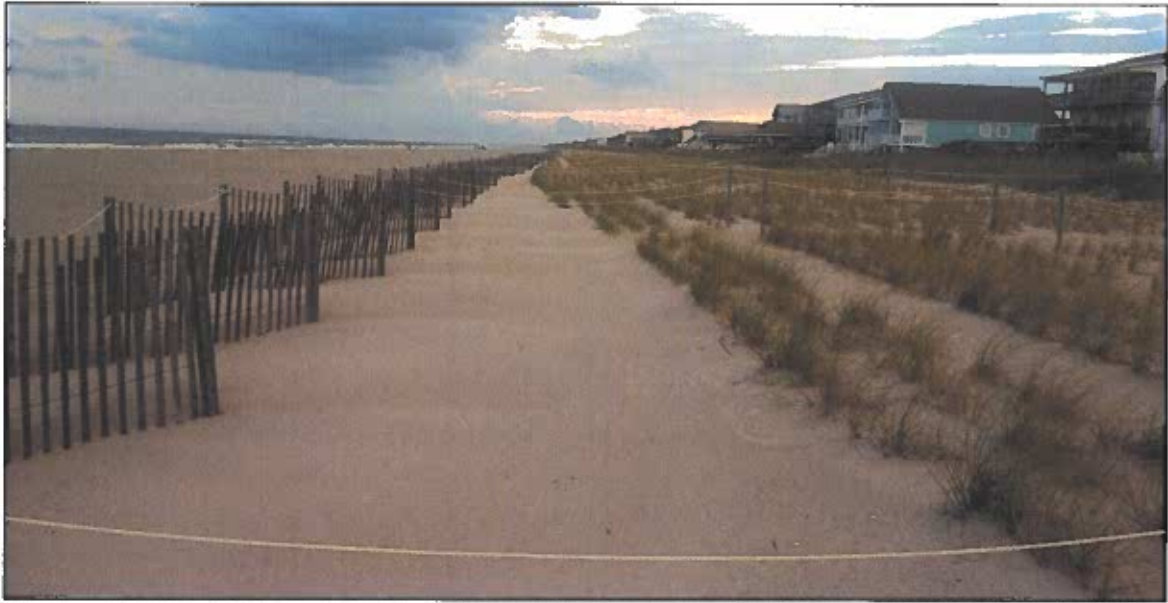
Figure 2-11 (B). Central Reach Post-Construction Approximately Station 230+00 (ATM photo taken August 2018). Note sand fencing, starter dune, and plantings.
