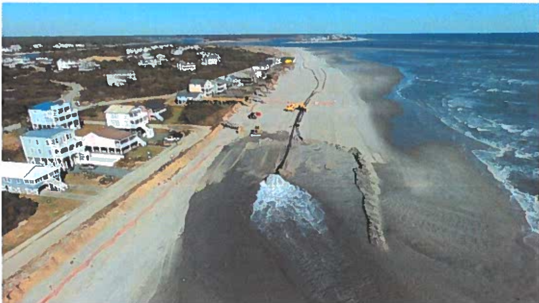
Figure 2-19. Holden Beach POA Aerial Photograph taken during 2017 Eastern Reach Project Construction (pumping just west of Station 30+00).
