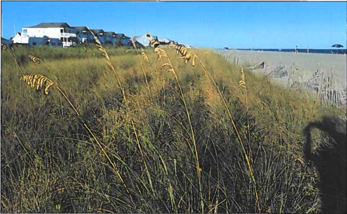
Figure 2-11 (F). Central Reach Post-Construction Approximately Station 170+00 looking east towards pier (ATM photo taken May 2020). Note plantings have matured and grown.
