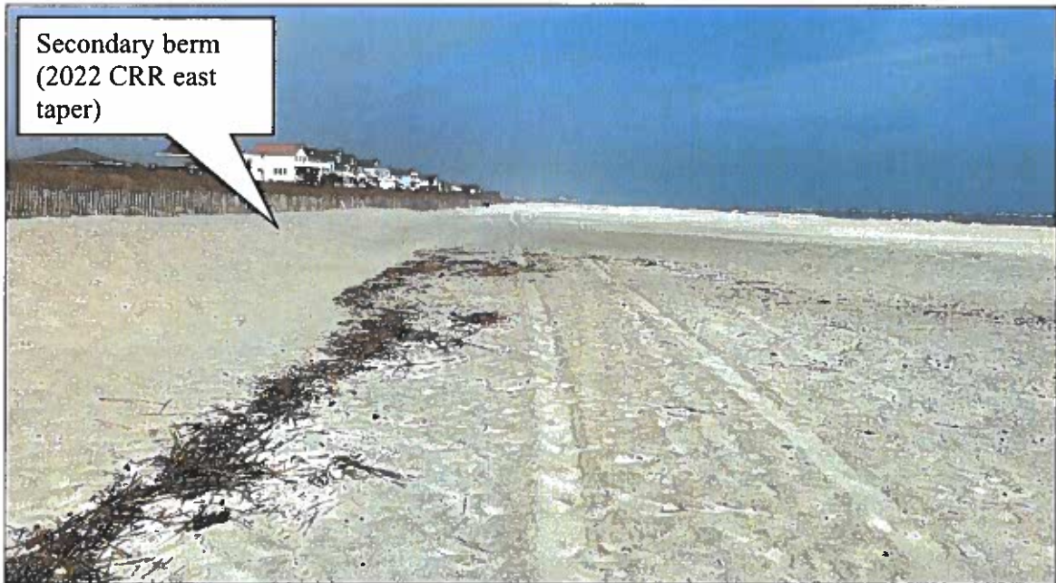
Figure 2-24 (B). April 2022 photograph near Station 40+00 looking east. Note newly constructed secondary berm along east taper of CRR which ties in with the 2022 LWFIX project at this location.
