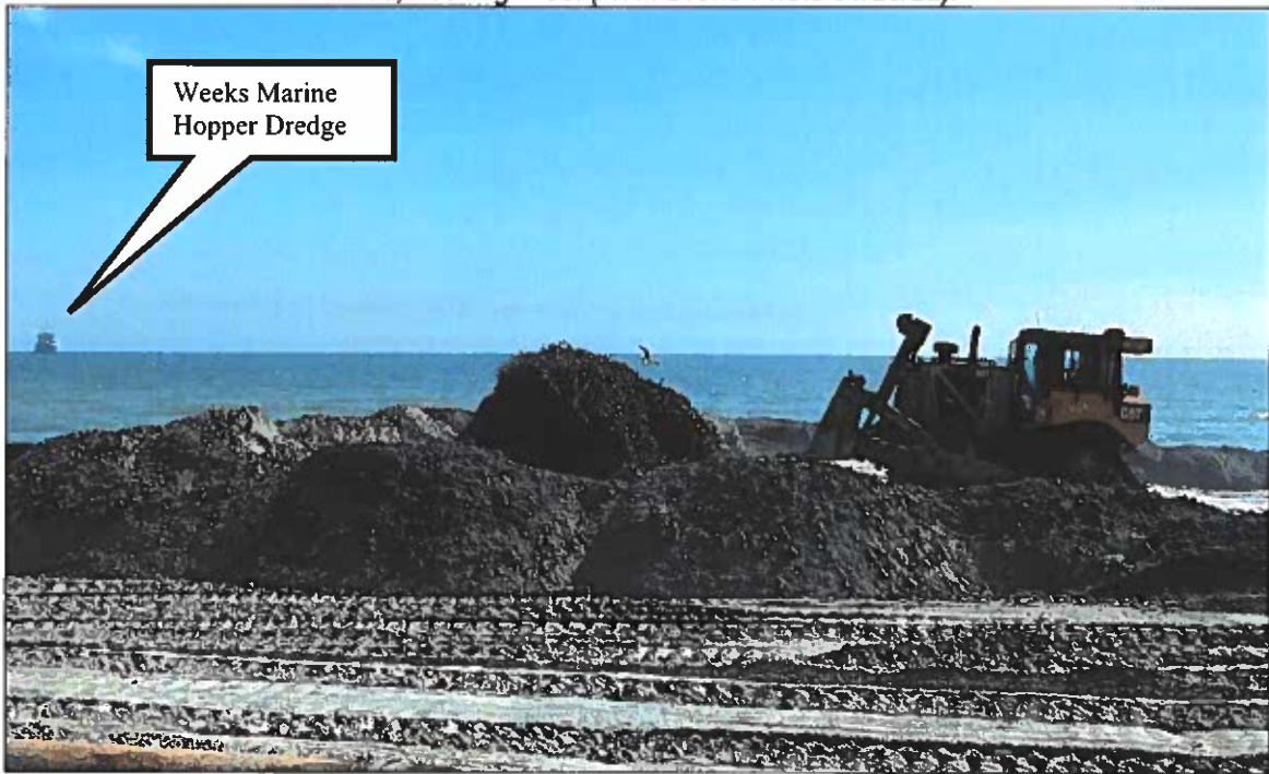
Figure 2-9 (B). CRR Construction Ground Photo (ATM photo taken 02/24/2022).
