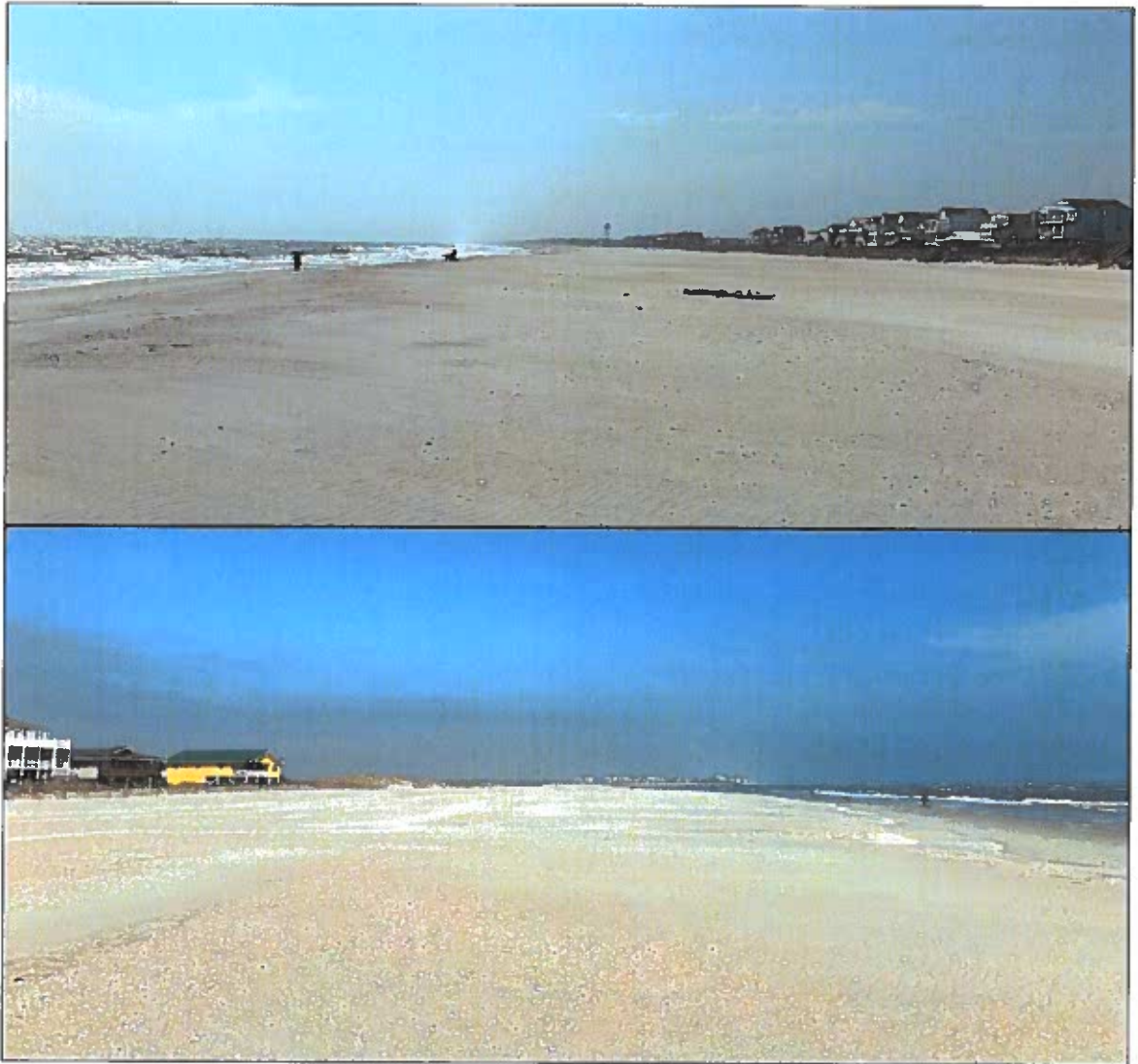
Figure 3-6. Recent Photograph of East End Beach Conditions Taken between Stations 20+00 and 30+00 Looking West (Upper Photo) and East (Lower Photo). 2022 LWIFX Placement Showing Wide Beach Present in What Is Typically an Erosional Hotspot Area (Photos Taken April 2022).
