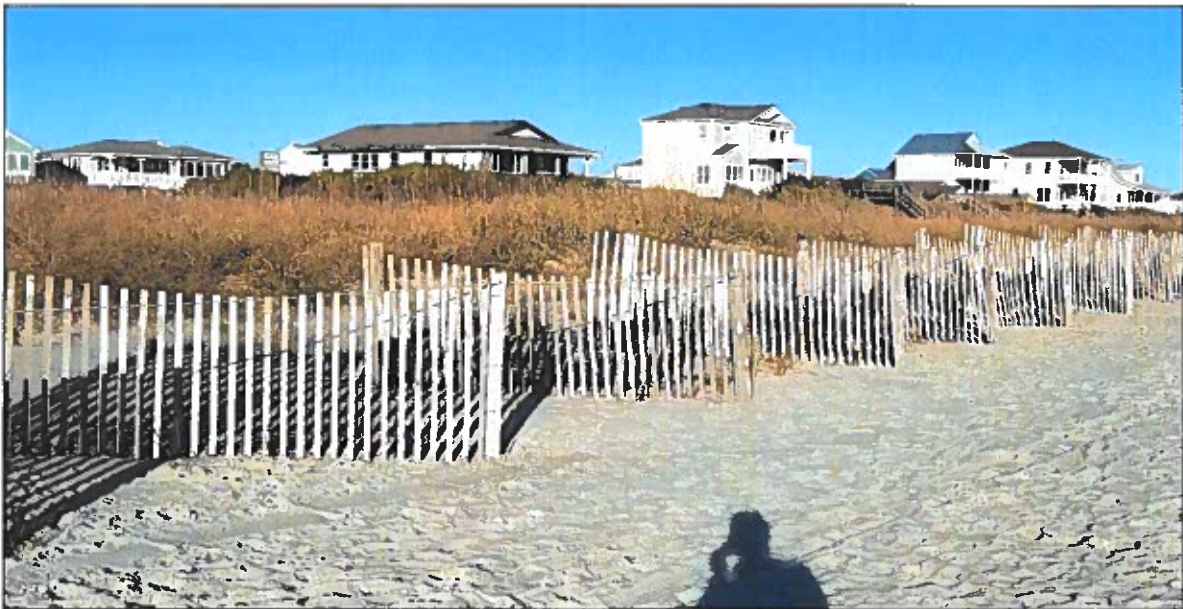
Figure 2-28 (D). November 2021 Station 60+00 after Hurricane Isaias which created some dune losses
