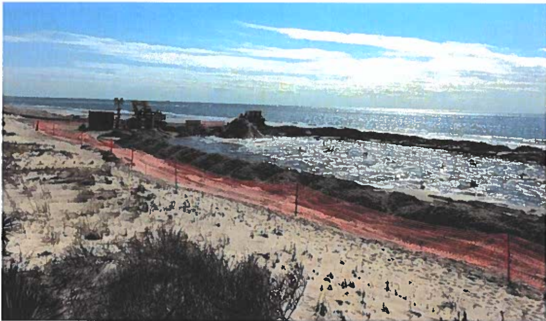
Figure 2-15. Holden Beach POA Photograph Taken near 323 McCray Street (approximately Station 26+00) during 2017 Eastern Reach Project construction.
