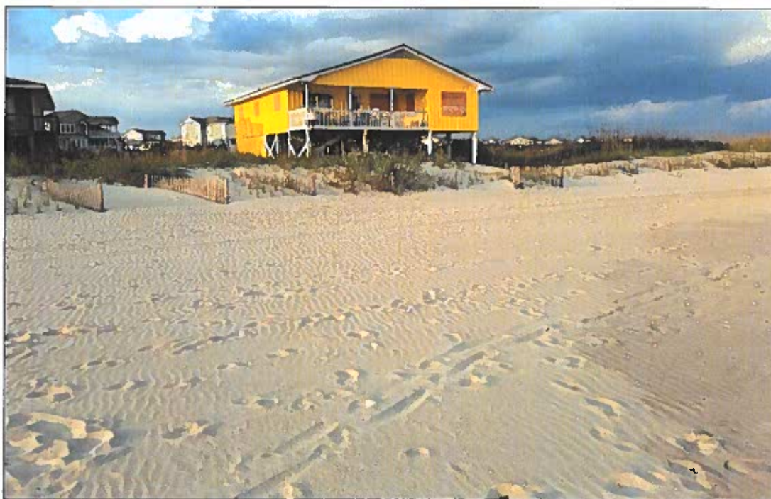
Figure 2-17. Two-Year Post Construction Photo of the 2017 Eastern Reach Project (ATM photo taken April 2018, at Station 20+00). The most eastern oceanfront house, Amazing Grace, is shown. Dune growth has occurred however this is still a vulnerable area.
