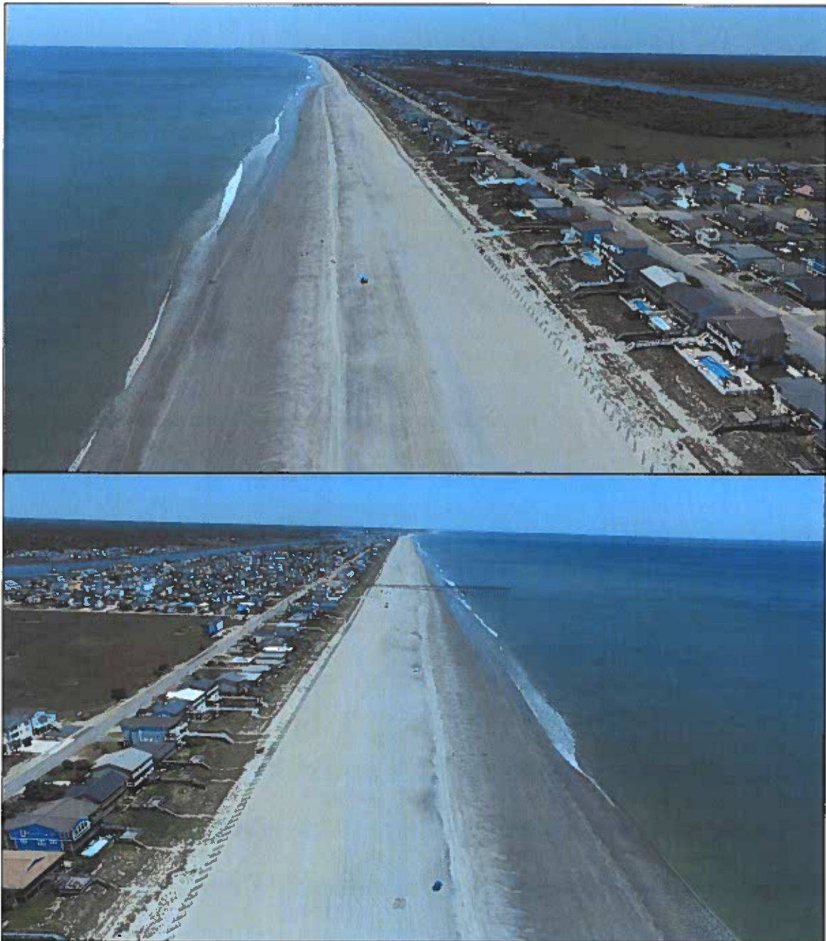
Figure 3-8. Central Reach April 2022 Aerial Photos Taken Near Station 200+00 Looking West Towards Shallotte Inlet in Upper Panel and East Towards the Pier and LWF Inlet in the Lower Panel.
