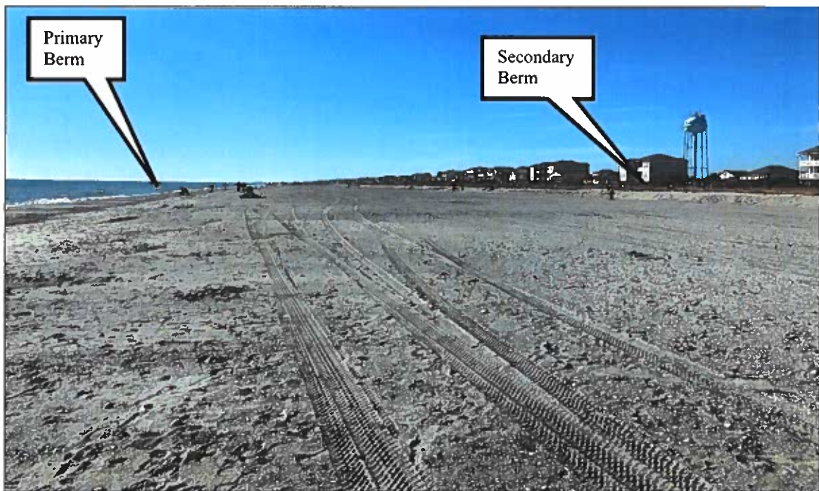
Figure 2-11 (A). CRR Post-Construction Near Station 80+00 (ATM photo taken 02/10/2022).
