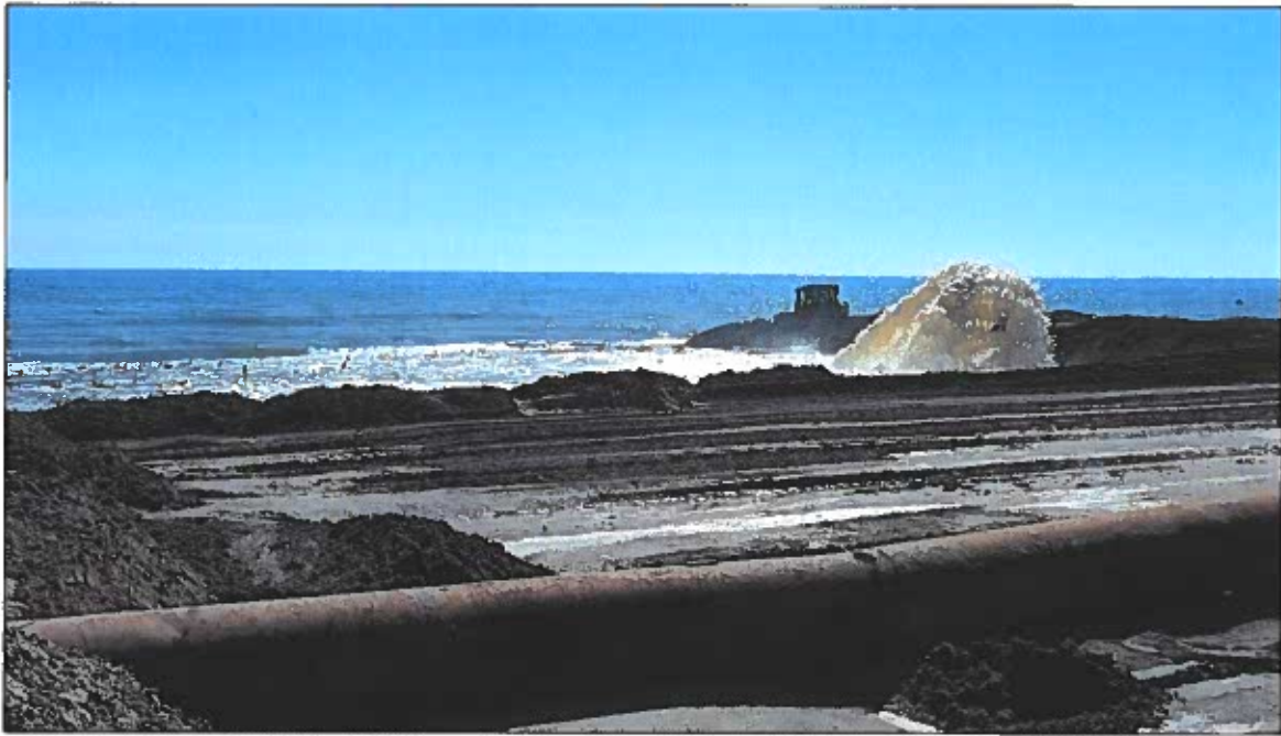
Figure 2-9 (C). CRR Construction Ground Photo (ATM photo taken 03/03/2022).
