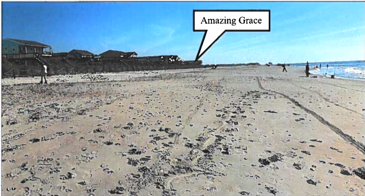
Figure 2-21 (D). October 2021 photograph near Station 30+00 looking East.
