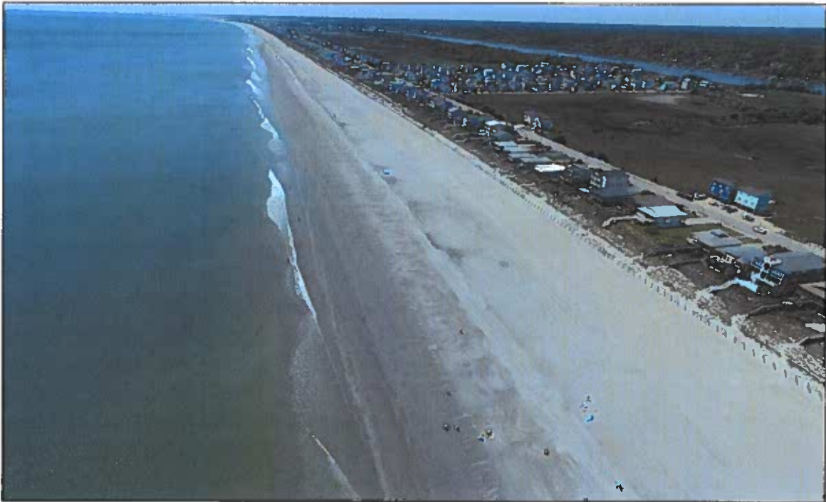
Figure 2-11 (B). CRR Post-Construction Aerial Photograph Taken Near Pier looking west (ATM photo taken 04/28/2022).
