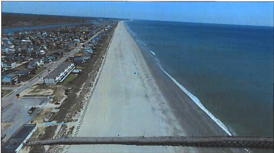
Figure 2-11 (C). CRR Post-Construction Aerial Photograph Taken Near Pier looking east (ATM photo taken 04/28/2022).
