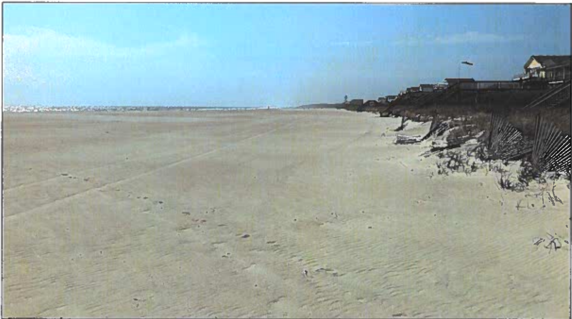
Figure 2-24 (C). April 2022 photograph taken between Station 20+00 and Station 30+00 looking west showing newly constructed 2022 LWFIX beach fill.
