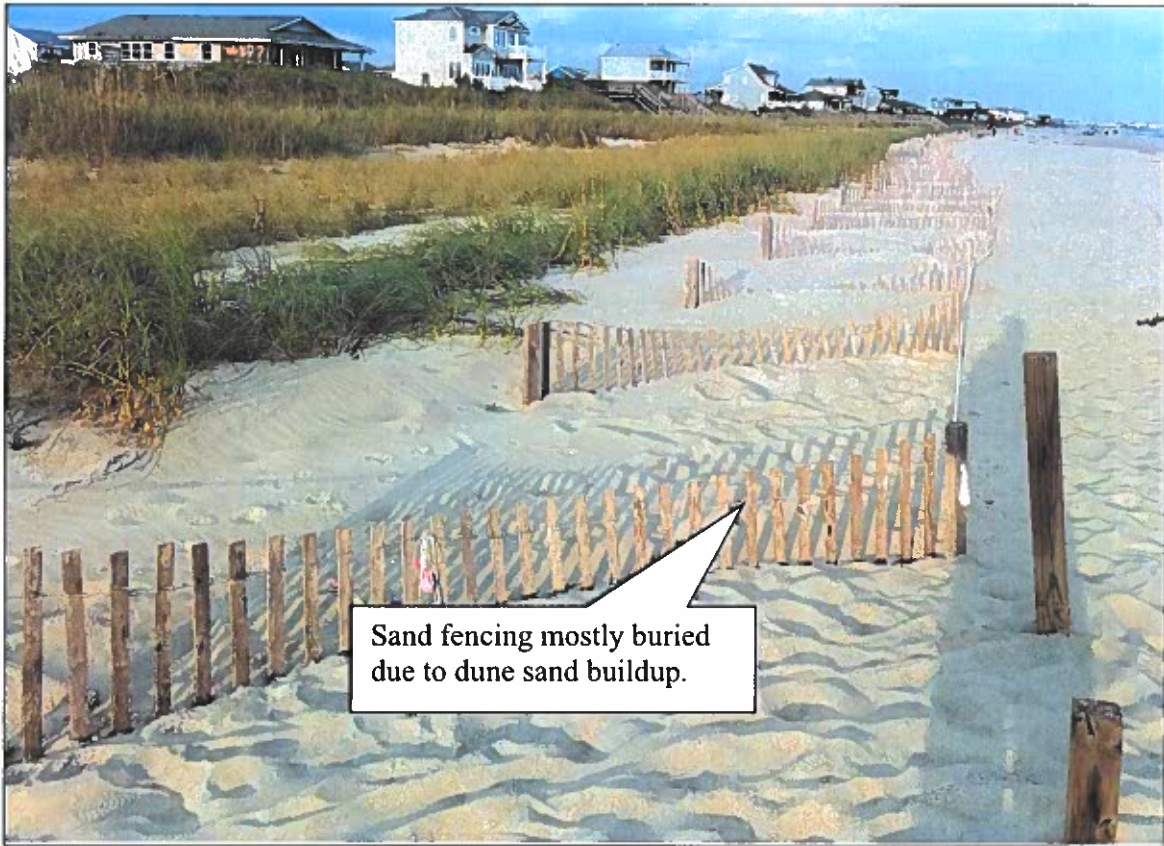
Figure 2-28 (B). Sand Fencing for the Central Reach Project at Station 60+00 showing dune vegetation and sand growth about 2-years post project. (ATM photo, taken September 2019).
