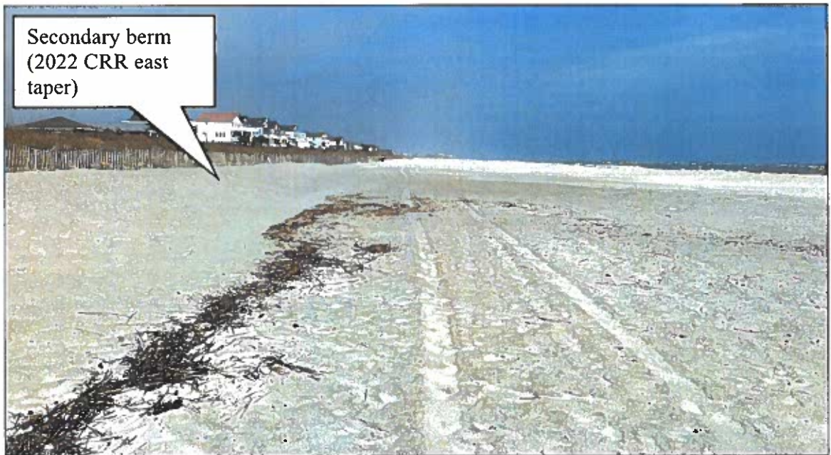
Figure 2-23 (B). April 2022 photograph near Station 40+00 looking east. Note newly constructed secondary berm along east taper of CRR which ties in with the 2022 LWFIX project at this location.
