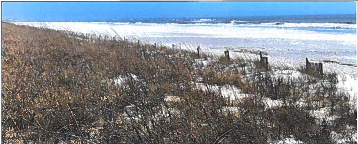
Figure 2-23 (A). April 2022 upland photograph taken near Station 40+00 showing healthy dune vegetation and wide beach following 2022 LWFIX construction.
