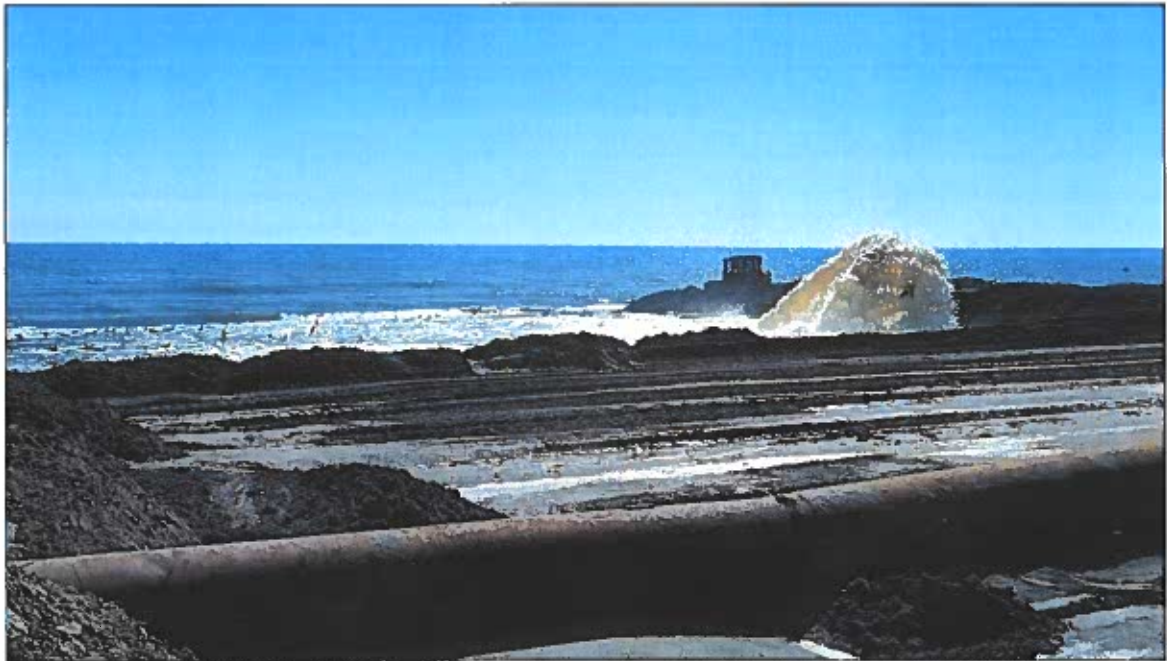
Figure 2-7 (C). CRR Construction Ground Photo (ATM photo taken 03/03/2022).
