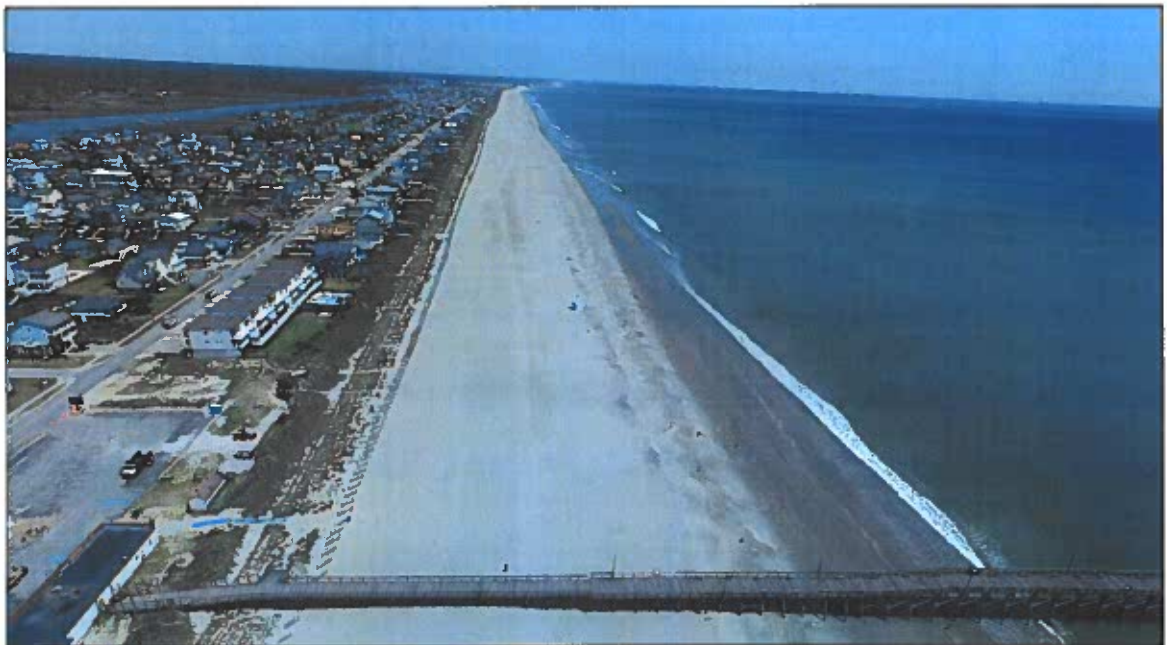
Figure 2-9 (C). CRR Post-Construction Aerial Photograph Taken Near Pier looking east (ATM photo taken 04/28/2022).
