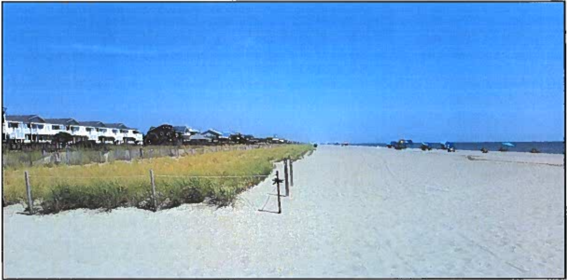
Figure 2-11 (A). CRR ~1.5 Year Post-Construction Photo Just East of Pier Near Station 170+00 (photo taken September 2023).
