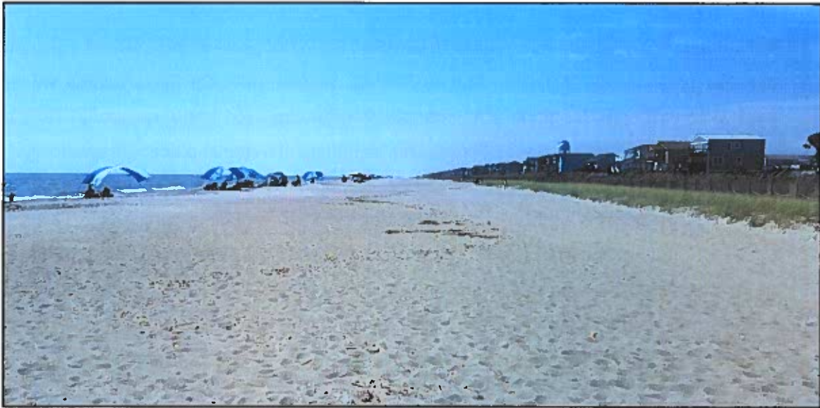
Figure 2-11 (C). CRR ~1.5 Year Post-Construction Photo Near Station 60+00 (photo taken September 2023).
