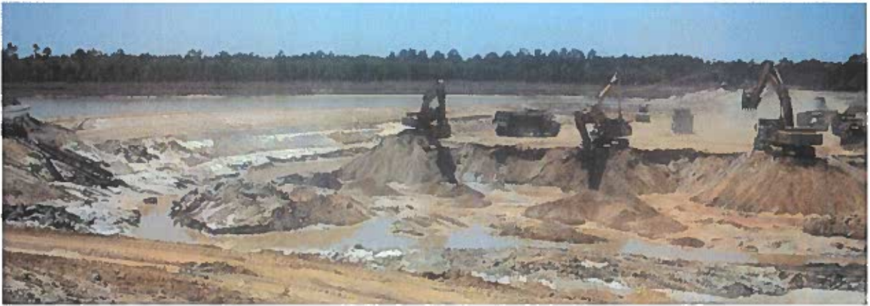
Figure 2-3. Smith Upland Borrow Area during 2009 Holden Beach Nourishment Project
