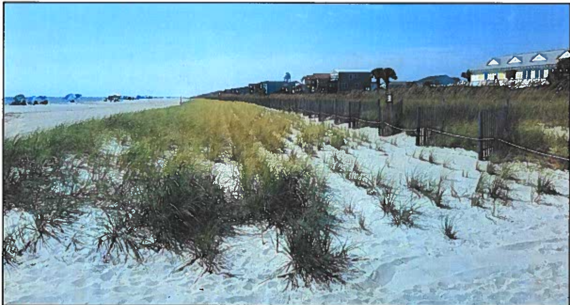
Figure 2-30. September 2023 between Station 60+00 and Station 70+00 showing plant growth ~1.5-year post CRR along newly constructed secondary berm (and after Hurricane Ian).
