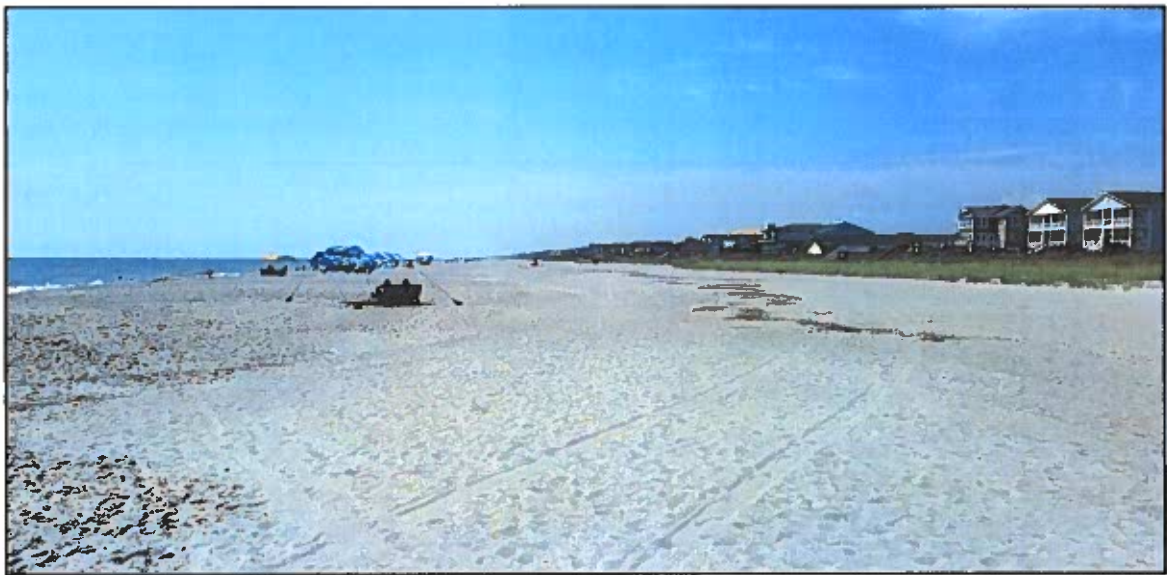
Figure 2-11 (B). CRR ~1.5 Year Post-Construction Photo Just West of Pier Near Station 170+00 (photo taken September 2023).
