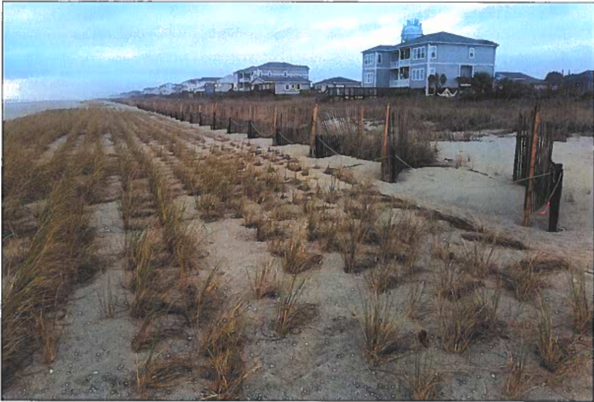
Figure 2-29. November 2022 near Station 80+00 showing new plantings following CRR along newly constructed secondary berm (and after Hurricane Ian).
