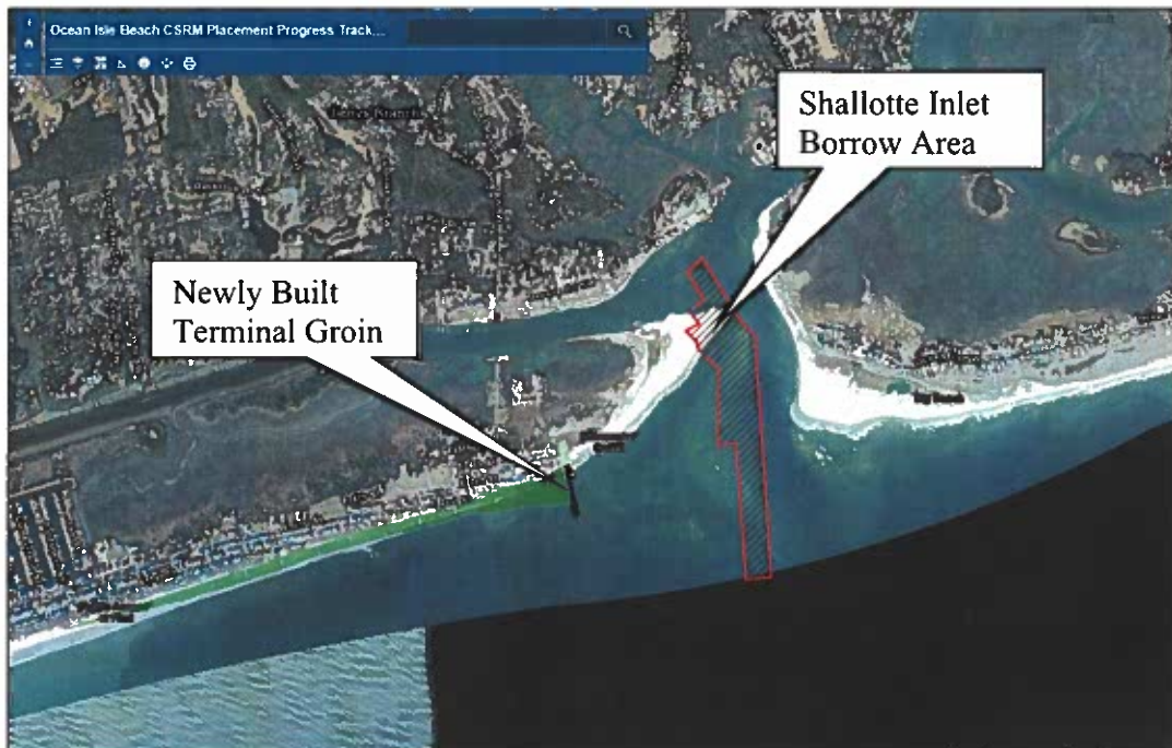
Figure 3-10. Ocean Isle Beach 2021/2022 Terminal Groin and Federal CSRM Beach Renourishment Projects. Shallotte Inlet Borrow Area and Placement Area Shown (USACE Ocean Isle Beach CSRM Placement Progress Tracker)
