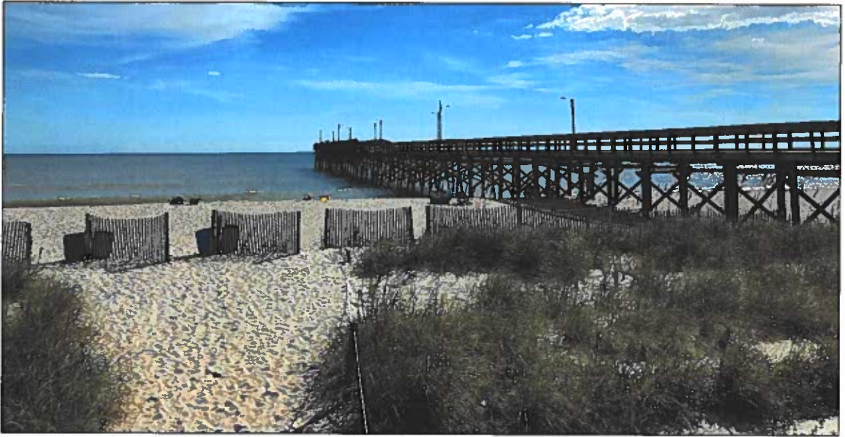
Figure 2-10 (B). October 2021 Photograph Taken Near Pier (~Station 170+00) Looking West.
