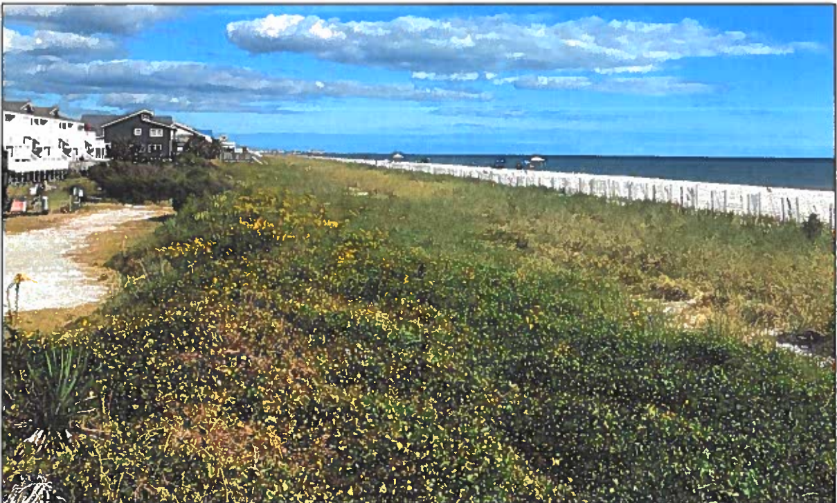
Figure 2-11 (G). Central Reach Post-Construction Approximately Station 170+00 looking east (ATM photo taken October 2021). Note plantings have matured and grown (right hand side of photo) and are overall healthy following damage from Hurricane Isaias in August of 2020.
