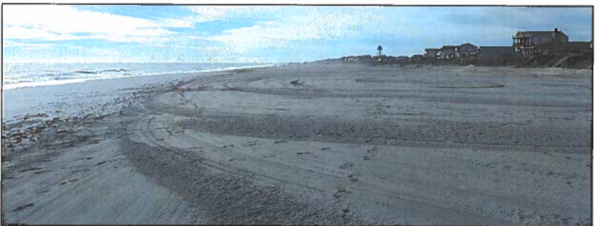
Figure 2-11 (A). Central Reach Immediate Post-Construction Approximately Station 50+00 (ATM photo taken January 2017)
