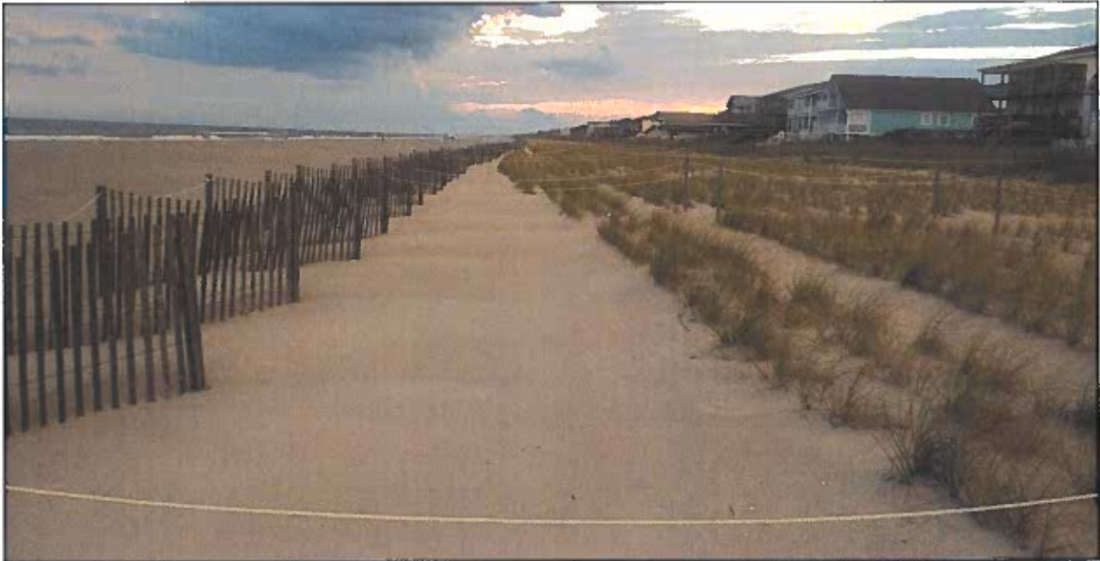
Figure 2-11 (B). Central Reach Post-Construction Approximately Station 230+00 (ATM photo taken August 2018). Note sand fencing, starter dune, and plantings.
