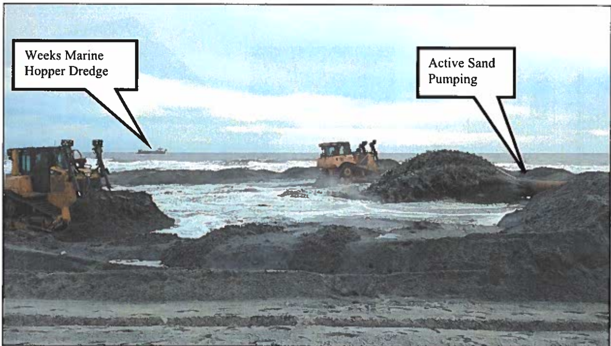
Figure 2-8. Central Reach Construction (ATM photo taken 1/26/17).
