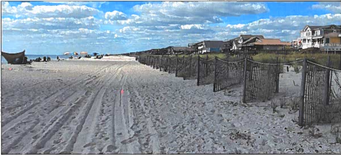
Figure 3-8 (B). Central Reach October 2021 Photo Taken Near Station 230+00 Looking East.
