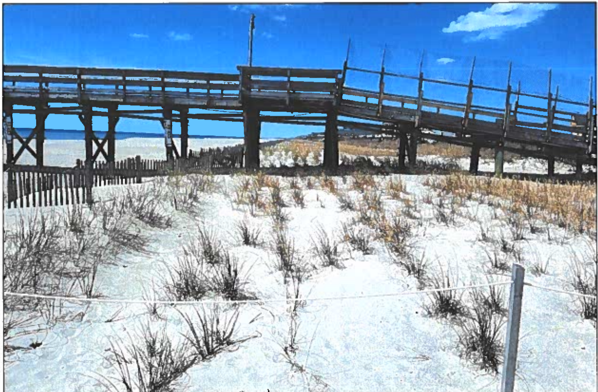
Figure 2-11 (C). Central Reach Post-Construction Approximately Station 170+00 (ATM photo taken March 2019).
