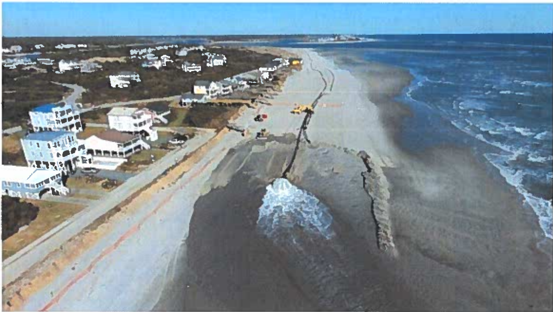
Figure 2-19. Holden Beach POA Aerial Photograph taken during 2017 Eastern Reach Project Construction (pumping just west of Station 30+00).
