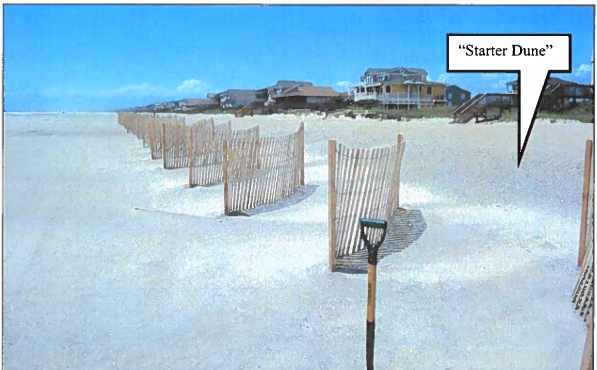
Figure 2-29 (B). Sand Fencing along the Seaward Edge of the Starter Dune for the Central Reach Project at Station ~230+00. Vegetation has been planted on the starter dune since photograph date. (ATM photo, taken May 2017).
