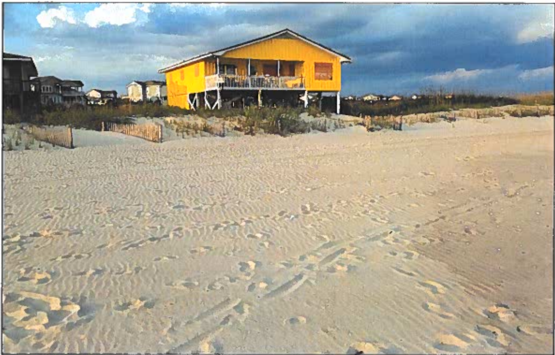
Figure 2-20. Two-Year Post Construction Photo of the 2017 Eastern Reach Project (ATM photo taken April 2018, at Station 20+00). The most eastern oceanfront house, Amazing Grace, is shown. Dune growth has occurred however this is still a vulnerable area.
