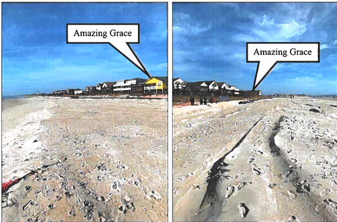
Figure 2-24 (a). Photograph in East End Taken During 2020 LWFIX Construction. (Holden Beach Town Newsletter)
