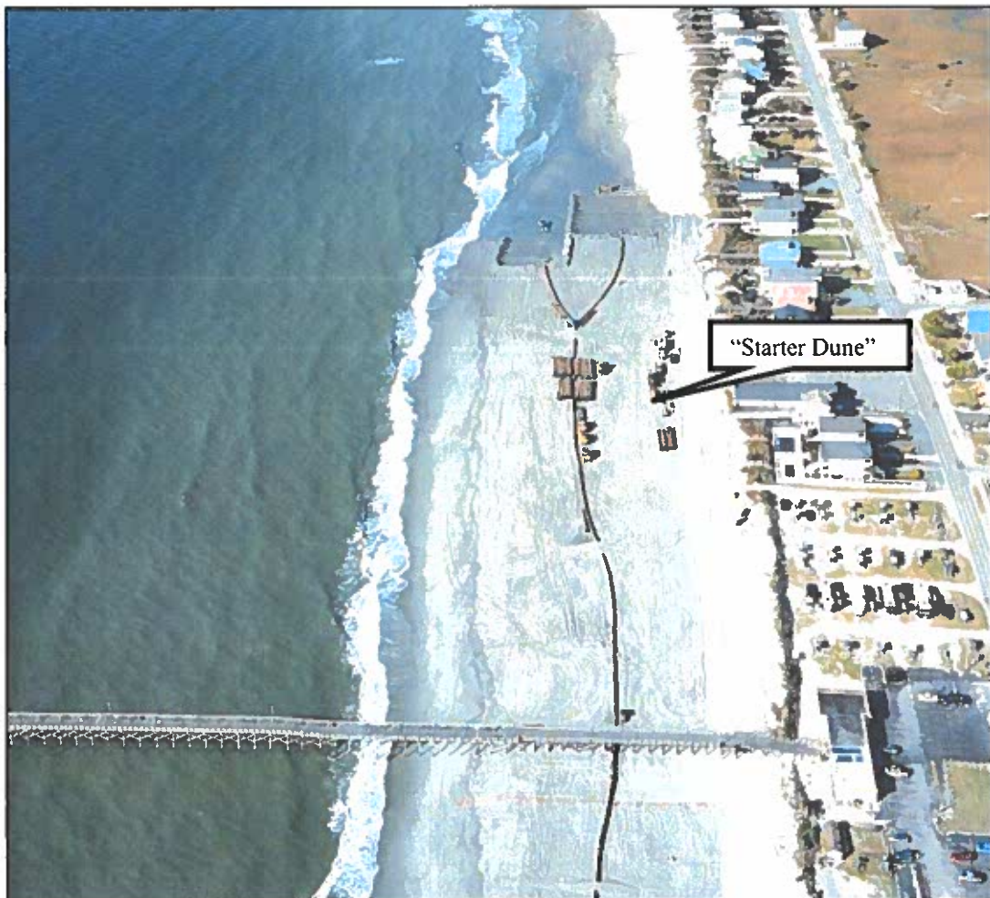
Figure 2-7. Aerial Photograph during Central Reach Construction West of Pier, Approximately Station 180+00 (Weeks Marine/Aerophoto Photo 2/22/17).
