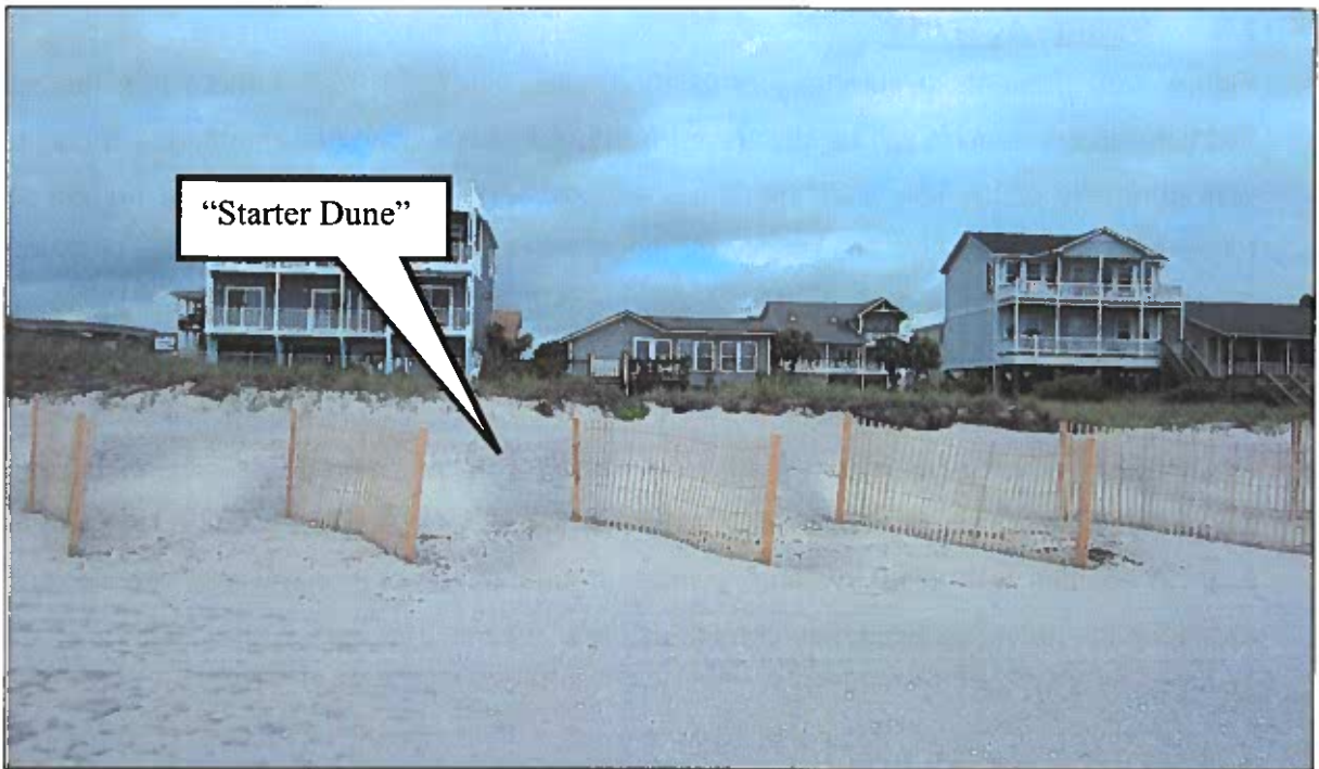
Figure 2-29 (A). Sand Fencing along the Seaward Edge of the Starter Dune for the Central Reach Project at Station ~60+00. Vegetation has been planted on the starter dune since photograph date. (ATM photo, taken May 2017).
