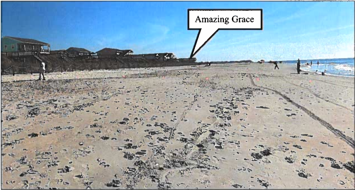
Figure 2-24 (d). October 2021 photograph near Station 30+00 looking East.
