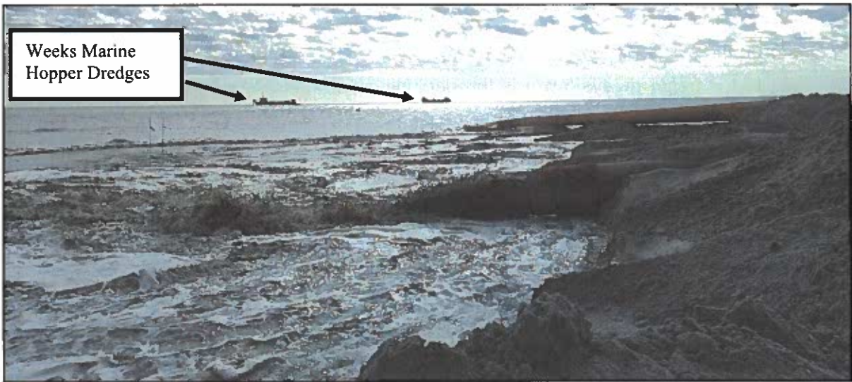
Figure 2-6. Central Reach Construction (ATM photo taken January 2017).
