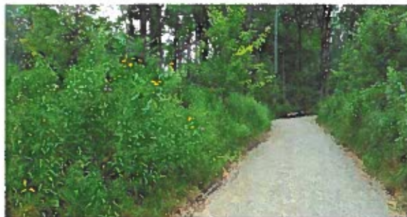
Natural surface trails are less expensive than asphalt paving and provide users with a pleasant walking experience.
