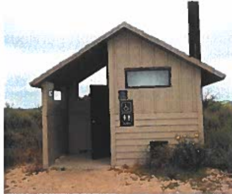
Example of waterless restroom
