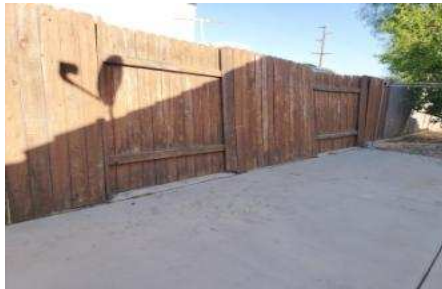
Loose/damaged fencing
