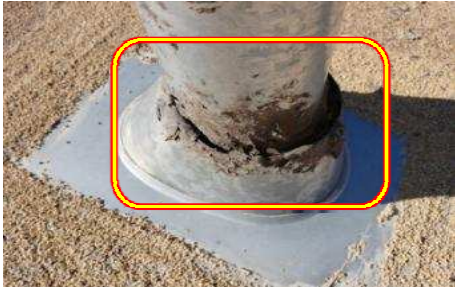
Weathered/missing sealant
