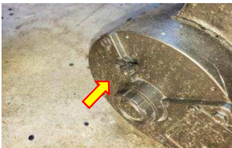
Bonding wire was missing
