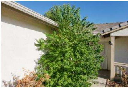
Vegetation was close to or in contact with structure
