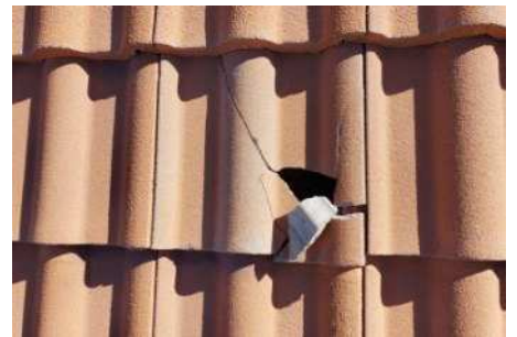
Damaged roofing tiles
