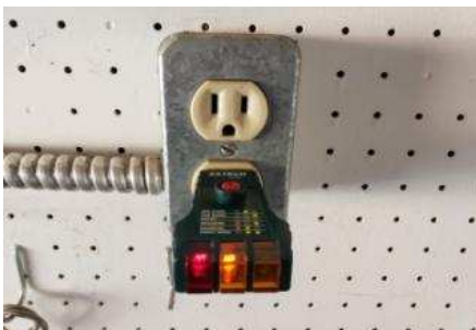
Reversed polarity outlet in garage
