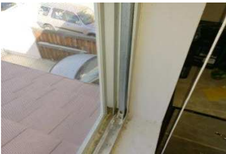
Damaged detached window balancers
