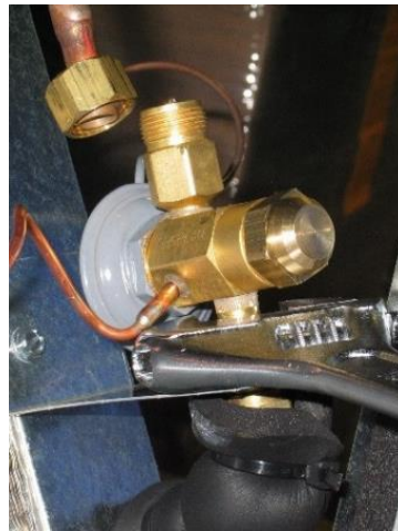
Figure 10 Attaching TXV to Distributor
