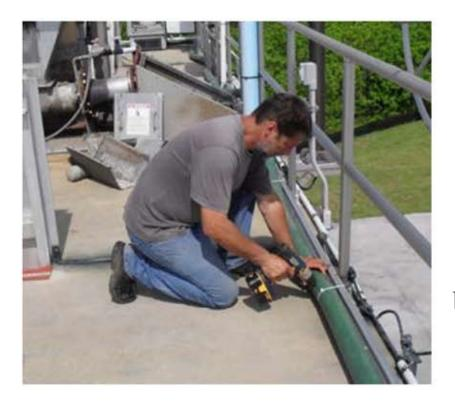
Secure hose with zipties and drill 1/4" diameter holes evenly spaced facing the odor source. Up to a maximum of 300 feet.
