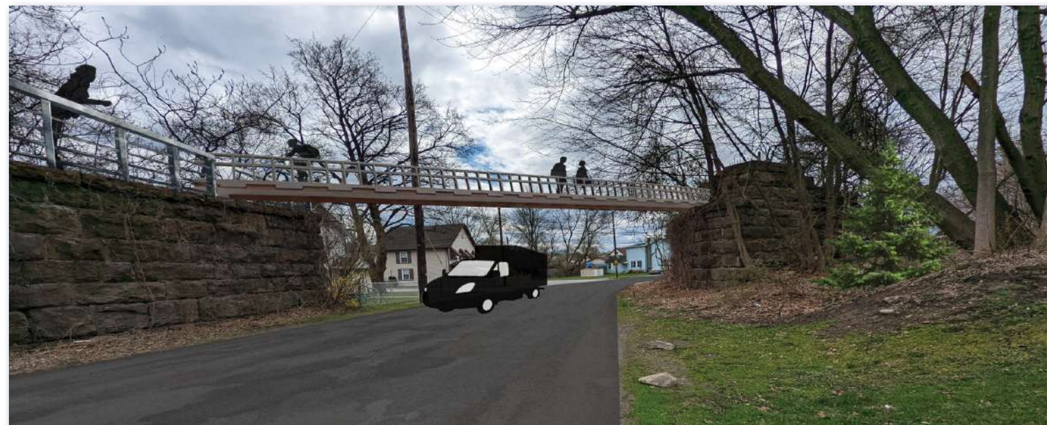
Trail crossing over Amelia Avenue. This area of The Plot will have two bridges that use remnant RR abutments and help to create a mini 'High-Line Park with green space on both sides of Amelia Avenue.
