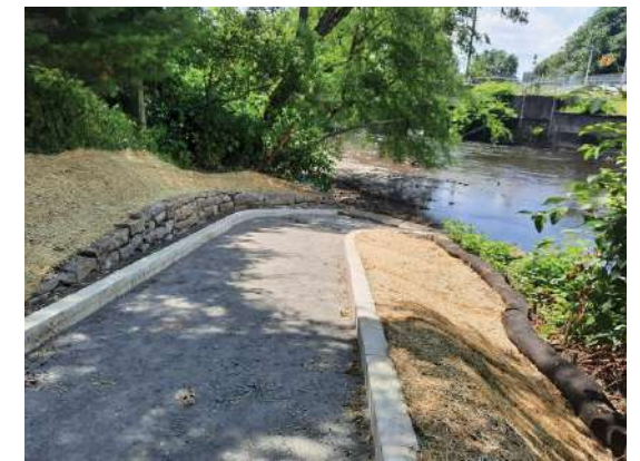
New j-hook fish habitat structure and an access ramp (under construction, July 2022)
