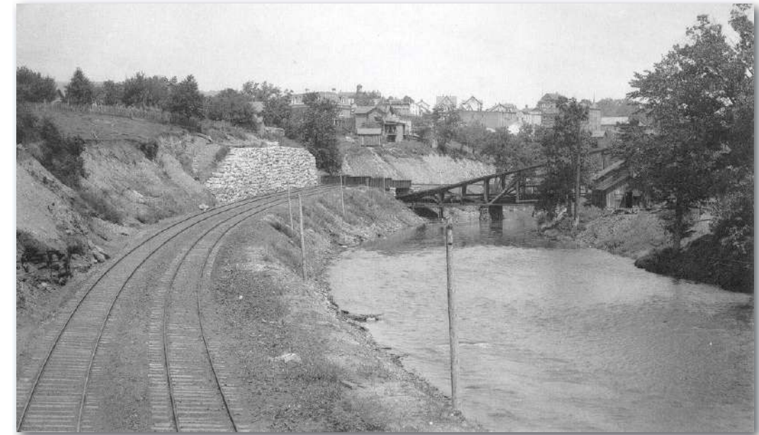
Looking north from Green Ridge Street; Historic photo shows the retaining wall and location where fill was placed behind Keen's.
