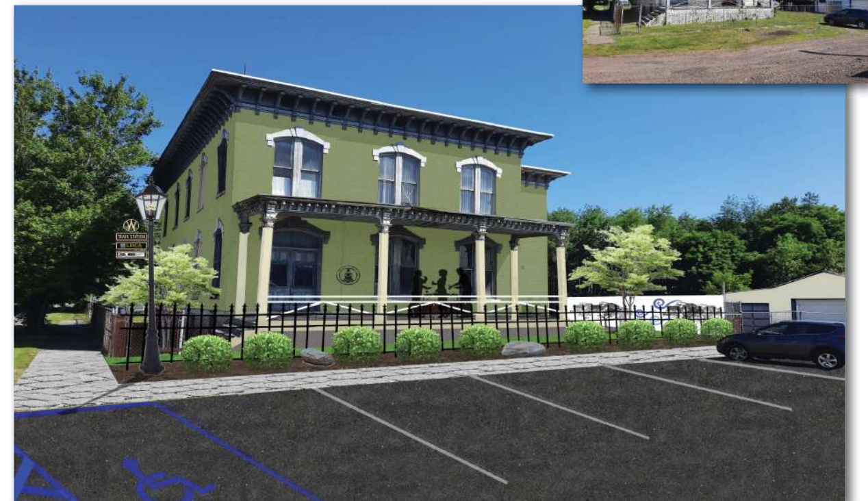
With the proper tenants and funders, the Depot building can undergo adaptive reuse as a restaurant/event venue/historic site and offices.
