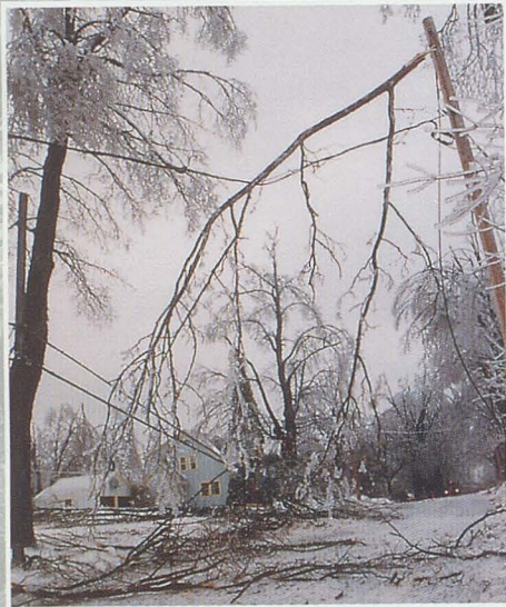
Roads were impassable due to downed trees and lines.
