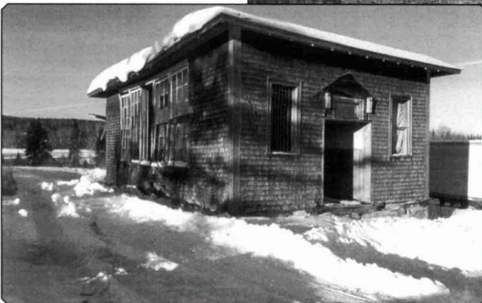
Longfellow School now waiting for the move.
