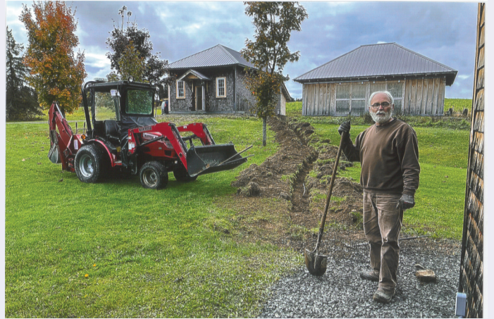
Dana Michaud digging the ditch to connect power to the school.
