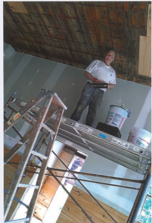
Jeff Trottier plastering the wall.
