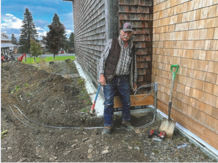
Gaylen Thibeault installing the electrical power to the school.
