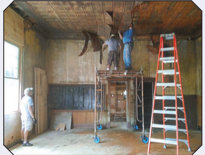
Messy job removing the old tin ceiling.
