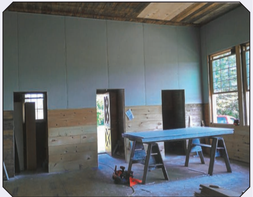
Dry wall installed.
