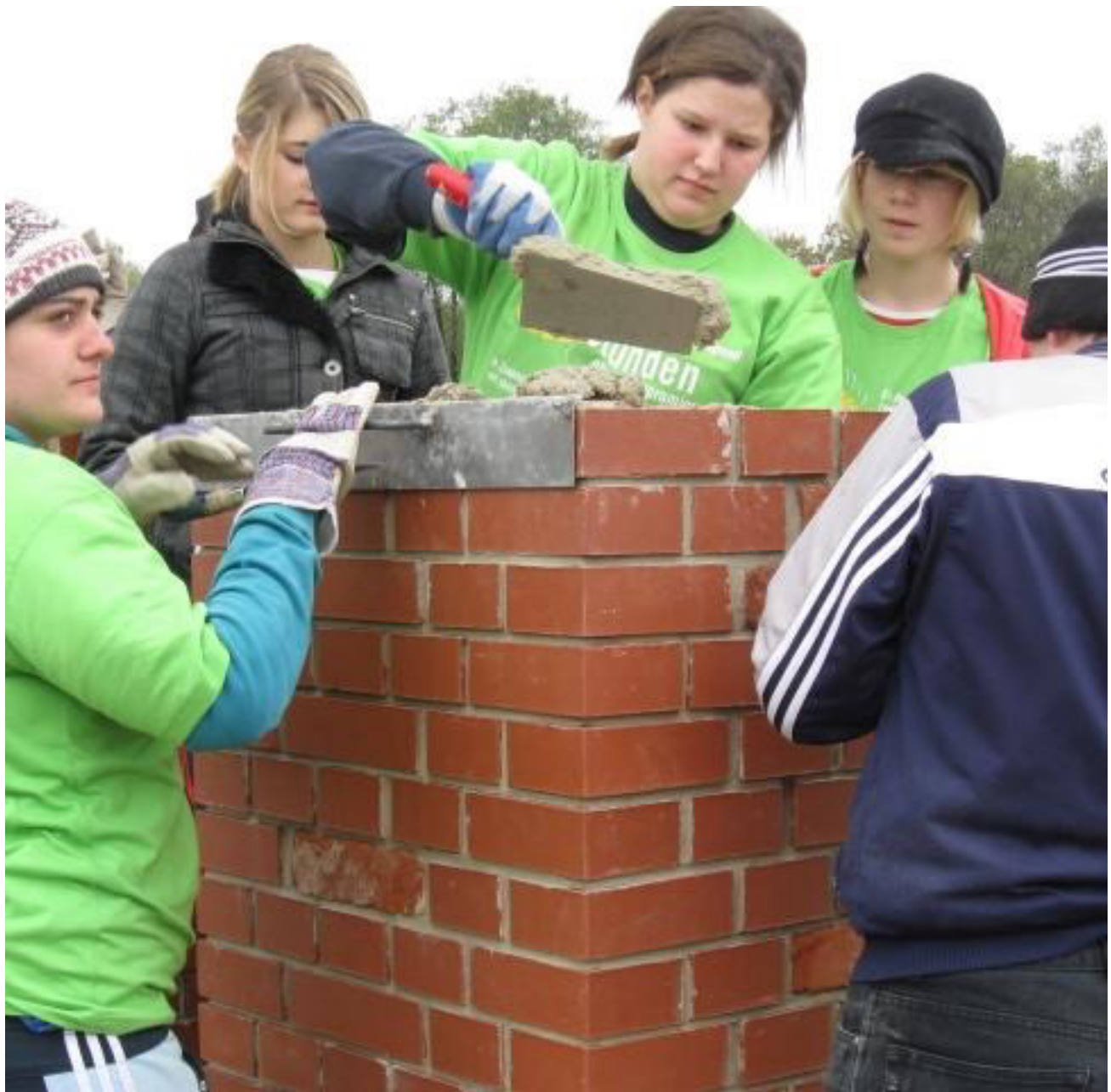
26. The 72 Hour Project is in progress.
