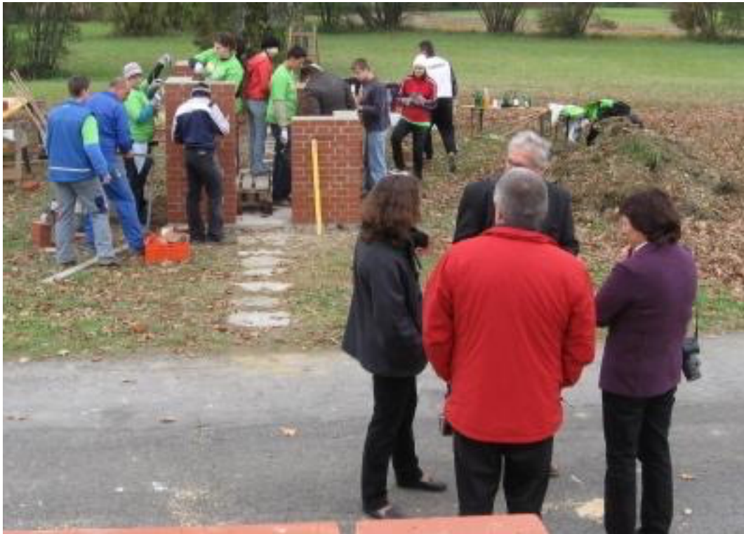
24. Friday (OCT 24, 2008) morning, visiting dignitaries at the 72 Hour Project site.
