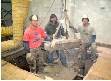
Pelland-Swenson working on the elevator shaft.
