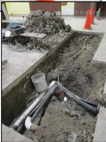
Photos of the boys locker room throughout the project
