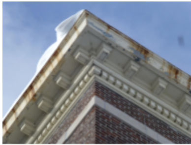
Photo 3 Location: Southeast corner Description: Typical cornice detail.
