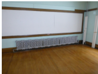
Photo 32 Location: Room 128 Description: Bank of few remaining original radiators.
