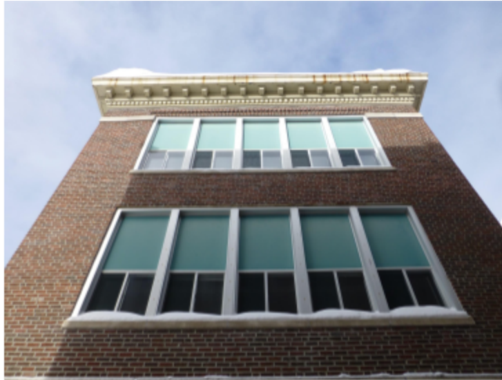
Photo 110 Location: southwest elevation Description: southwest corner of Baker building, Backus building just to the south.
