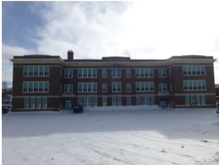
Photo 106 Location: north elevation Description: north elevation, significant snow cover on site at time of visit. Pavement extends to face of building.
