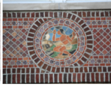
Photo 2 Location: North Elevation Description: Mosaic detail on north facade. Courtesy of Citizens for Backus/AB
