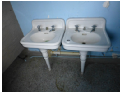
Photo 29 Location: Room 202 Description: Double pedestal sinks found in women's room 202 and 204 on level 2.
