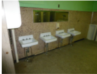
Photo 25 Location: Room 27 Description: Men's restroom at ground level showing replacement fixtures.
