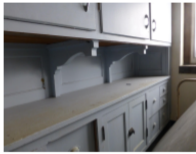
Photo 18 Location: Room 8 Description: Casework in room 8 on ground level. Original built-in casework with upper cabinet doors replaced.
