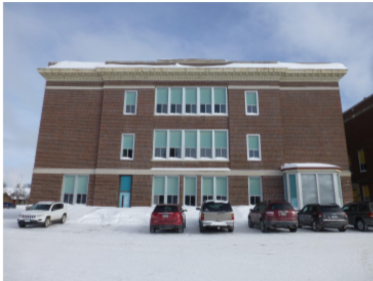
Photo 109 Location: west elevation Description: west elevation with single door and projecting conservatory at ground level,
