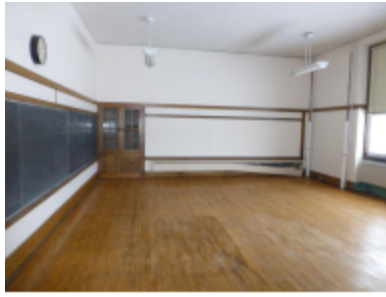
Photo 12 Location: Room 116 Description: Typical wood flooring in classroom.
