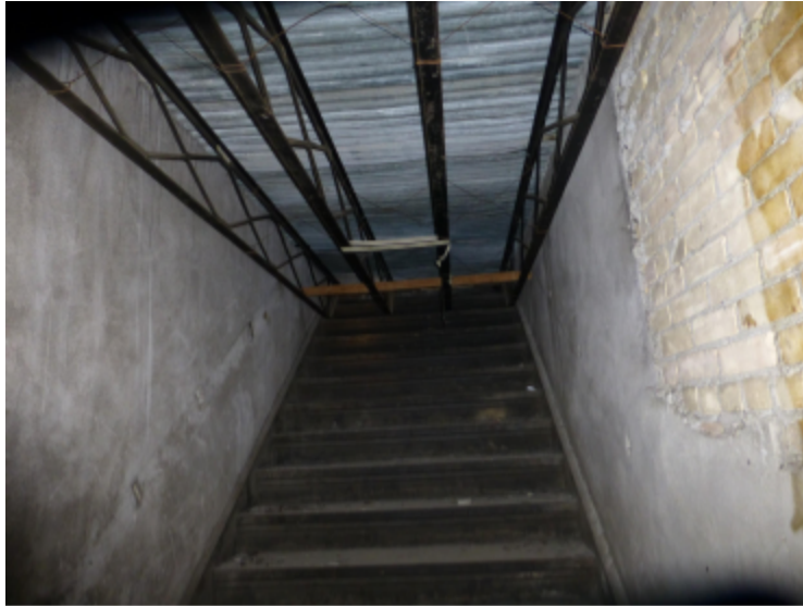
Photo 48 Location: Room B9 Description: Central stair to basement abandoned when Backus building was added.
