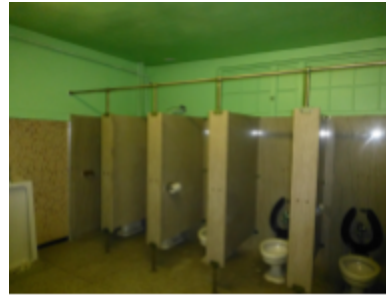
Photo 26 Location: Room 27 Description: Men's restroom on ground level original toilet partitions.
