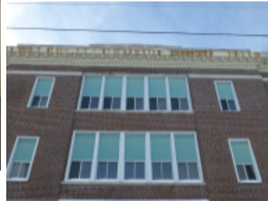
Photo 9 Location: East Elevation Description: Typical existing 1978 aluminum/insulated panel replacement windows
