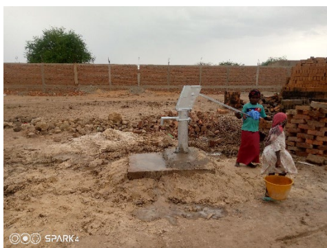
Borehole at completion
