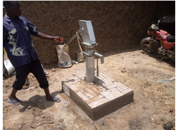
Dembe at completion
