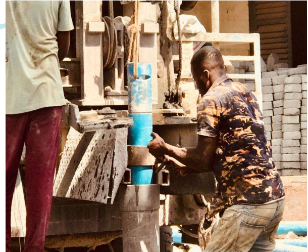
inserting the screen pipes
