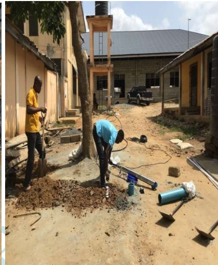
Fixing of Pump and electrical connection
