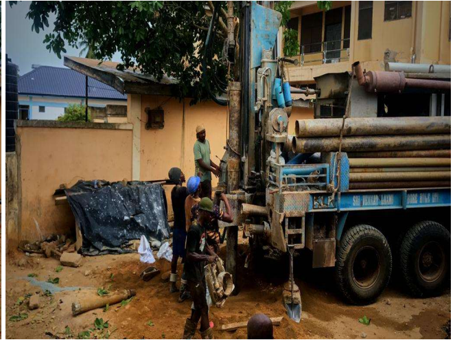
a. Positioning the drill barge in front of Boys Dormitory b. inserting steel pipe to shore surface overbearing
