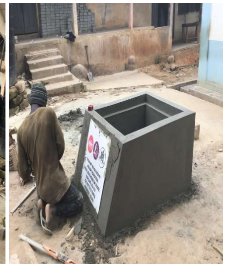
Construction of the chamber to house pump and dressing and fixing of plaque
