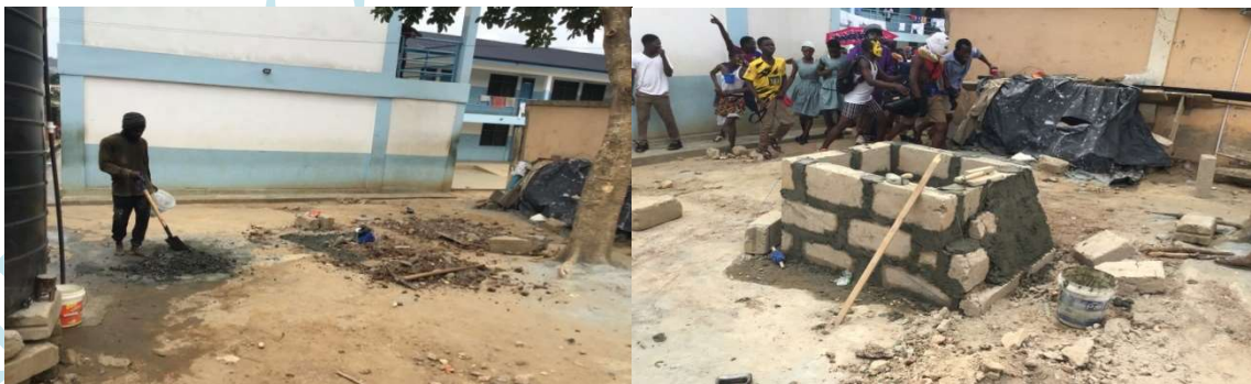
Construction of the Pump chamber
