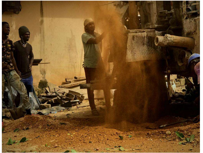
Drilling of well
