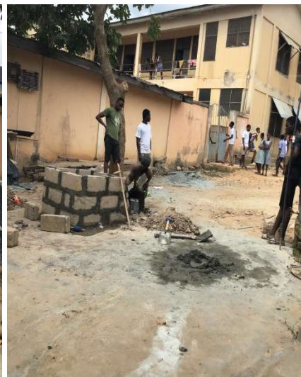
Construction of the chamber to house pump and dressing and fixing of plaque
