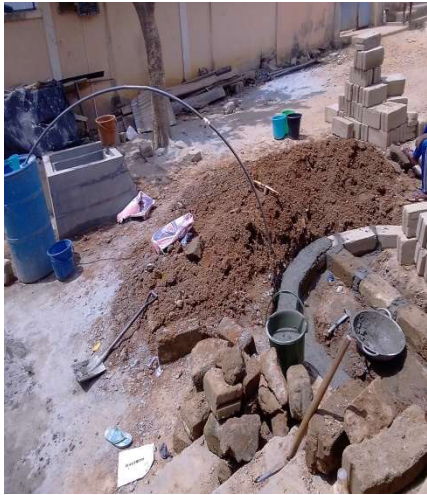
Construction of Poly tank platform
