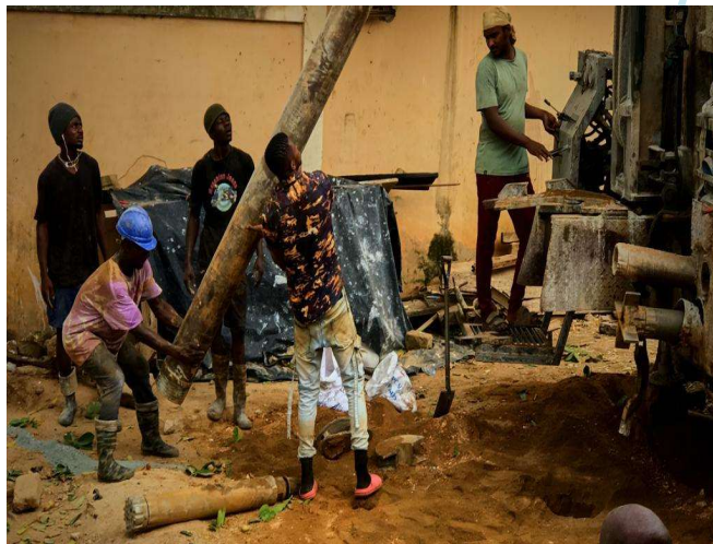
Removing the Steel casing
