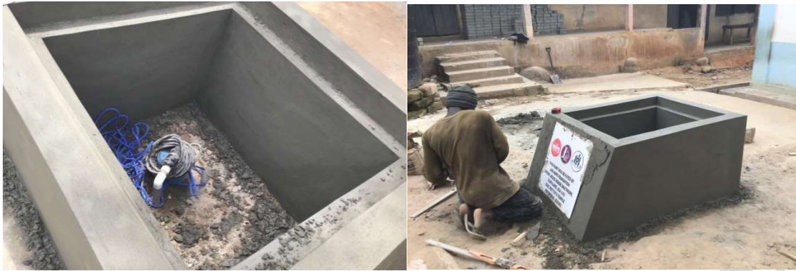
Construction of the Chamber
