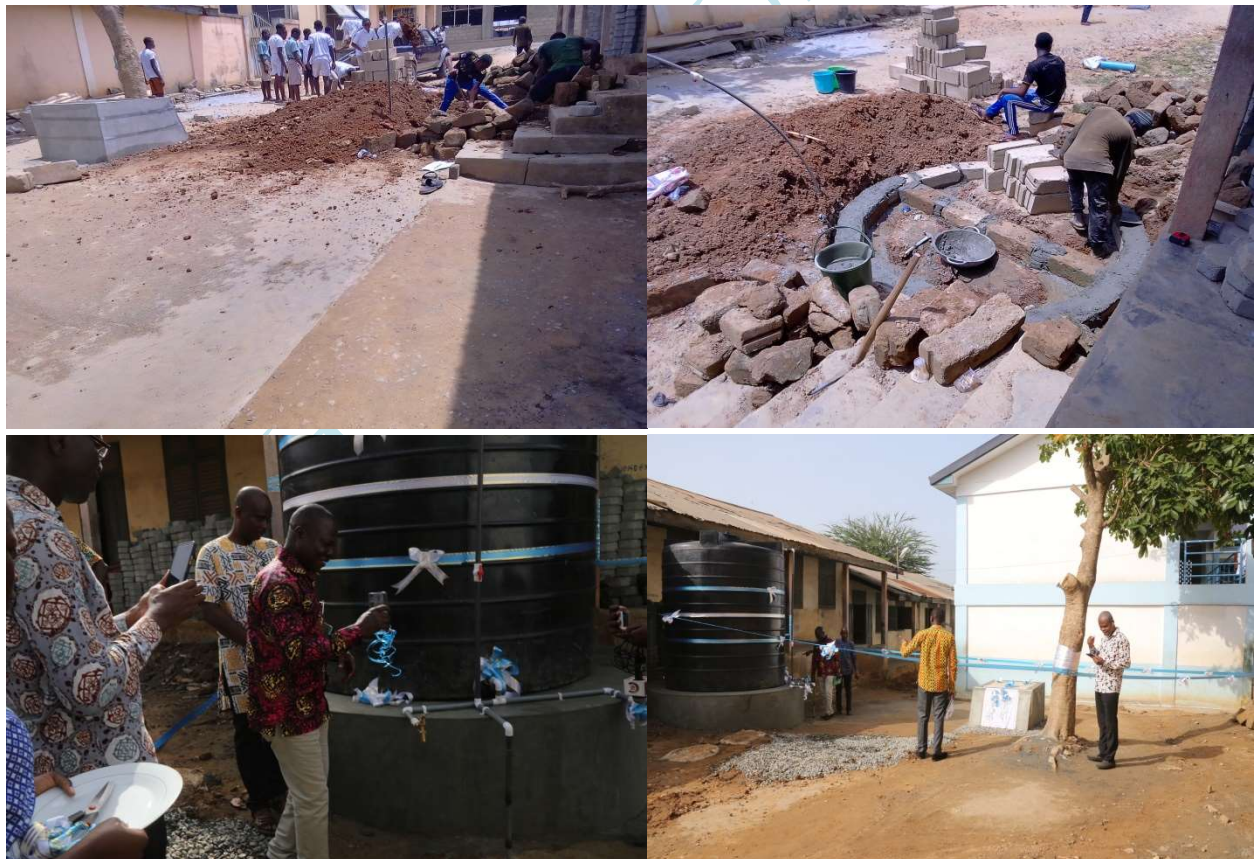
Construction of the Storage Platform
