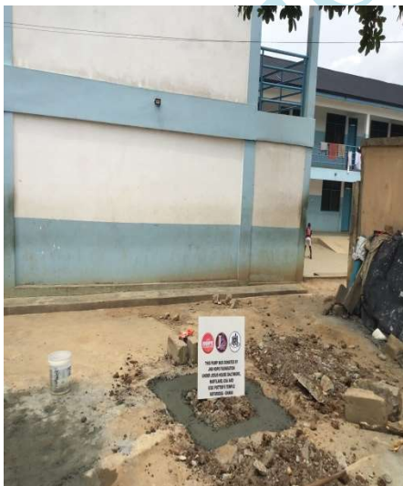
Construction of the chamber to house pump and dressing and fixing of plaque
