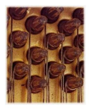
At the junction where rusted strings wrap around rusted pins, rust corrosion forms a hardened bond between the two. Then, during a tuning, when your piano technician turns the pins to stretch the strings, the inflexible, rusted string snaps at this joint.
