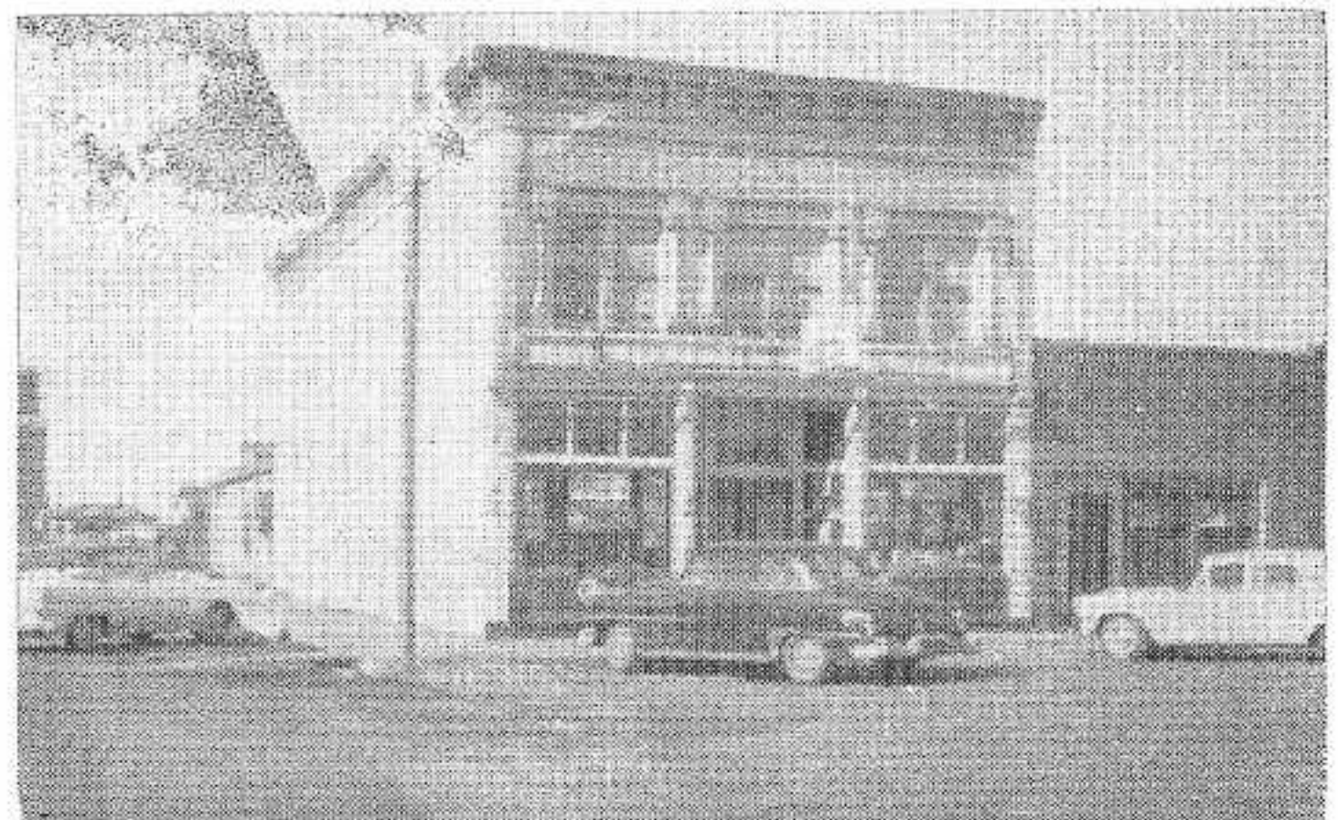
Present Store Building — 1947
