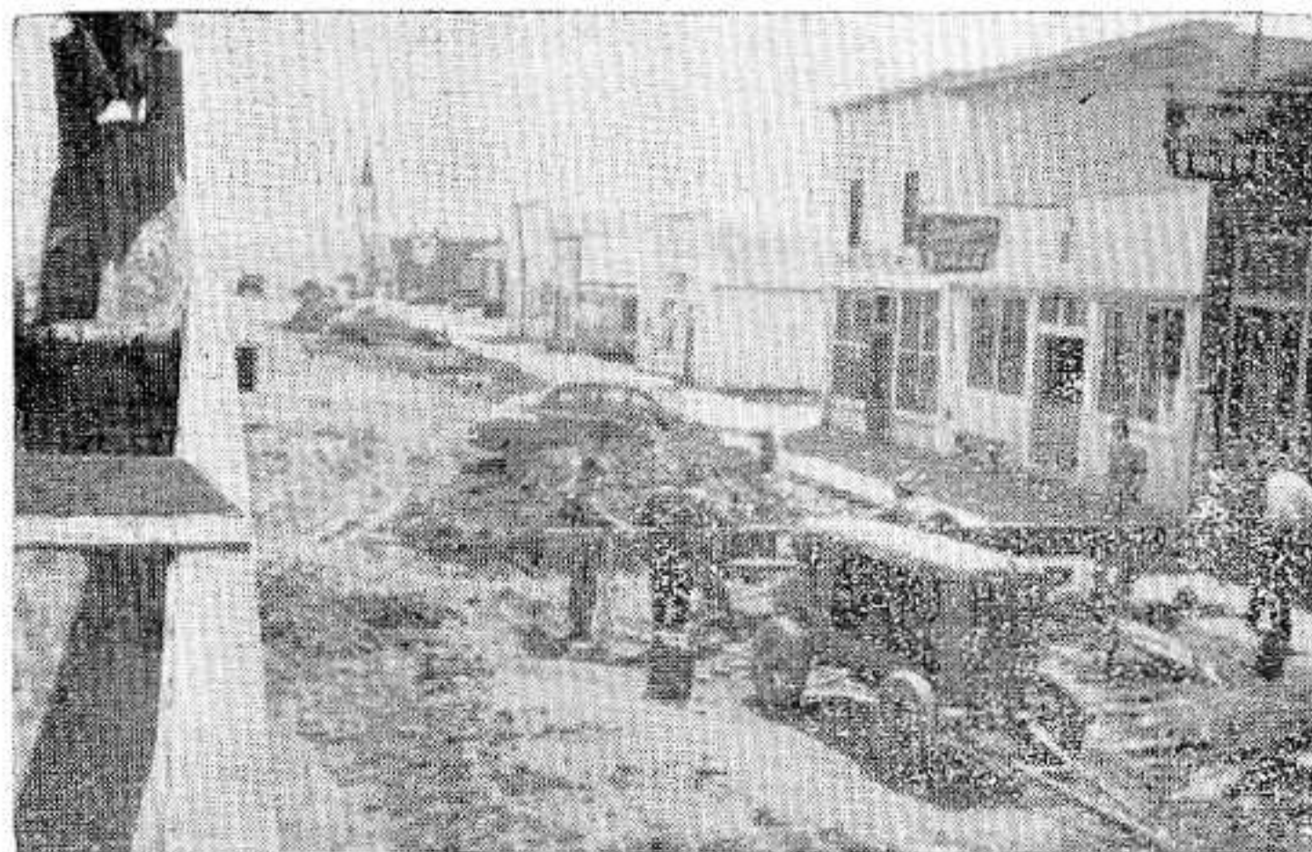
Putting in Sewer 1948, west side of main street
