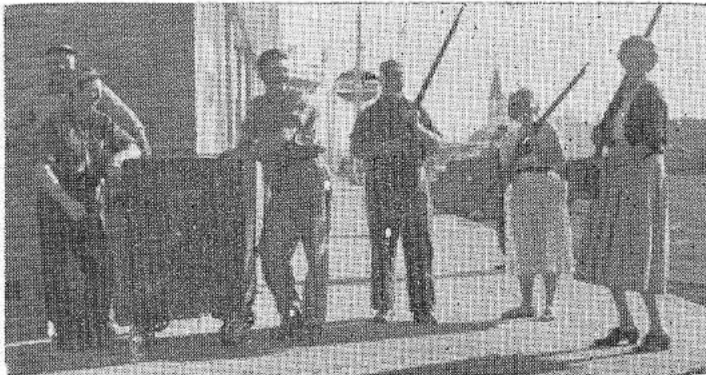
Moving to the new post office, 1958
