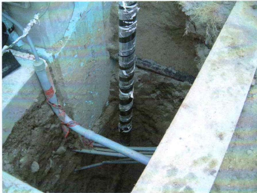
PHOTO #8 – Vertical forcemain excavation at consolidation building
