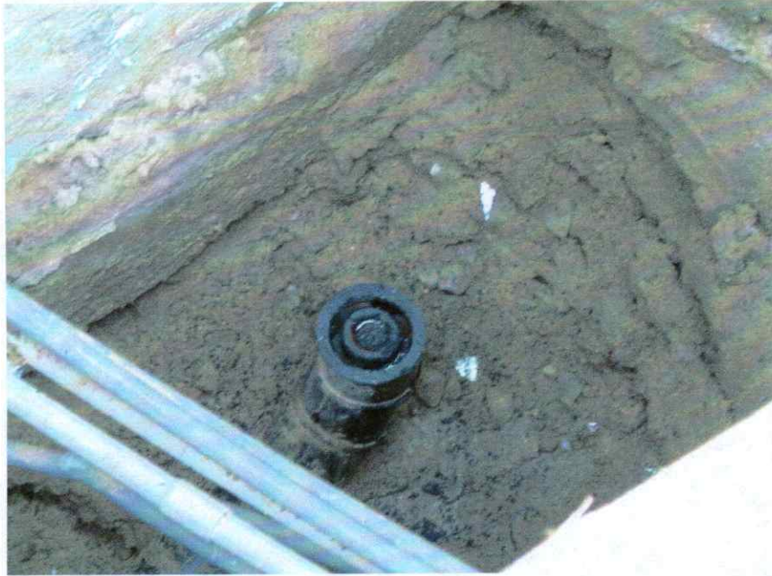
PHOTO #9 – 90° Elbow at bottom of vertical section of forcemain
