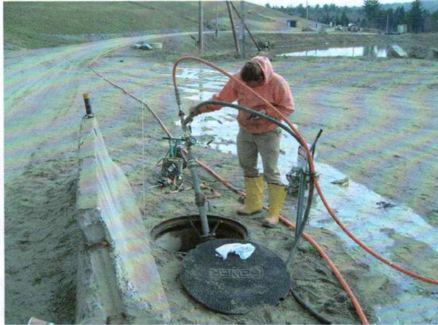
PHOTO #5 – Pneumatic testing of 4” carrier pipe at LMH-2
