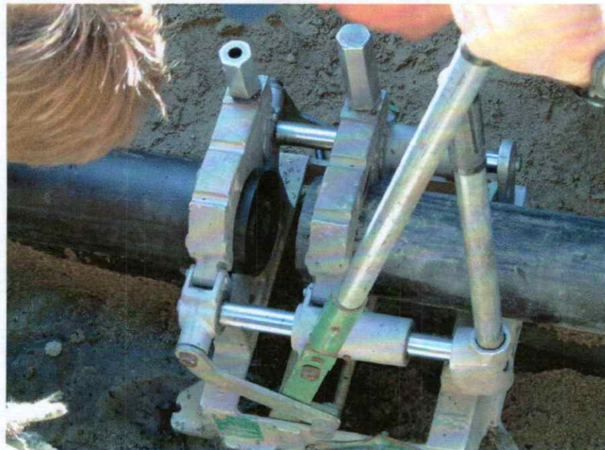
PHOTO #6 – Simulations butt-fusion welding of forcemain
