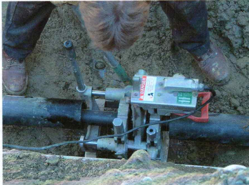
PHOTO #3 – Butt-fusion welding of 2" carrier pipe at Forcemain repair #1 location
