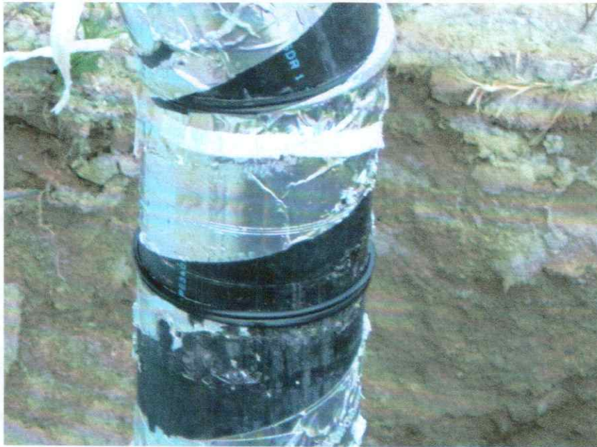
PHOTO #11 – Completed simultaneous weld in vertical section of force main
