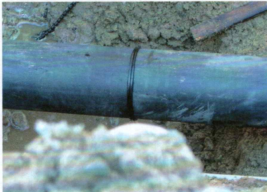
PHOTO #4 – Completed 4" containment pipe butt-fusion weld at Forcemain repair #1 location
