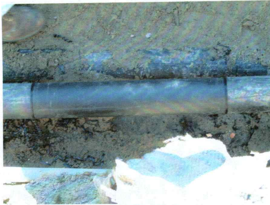
PHOTO #7 – Completed simultaneous butt-fusion weld
