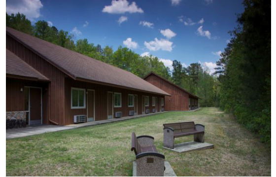
Retreat Center Buildings
