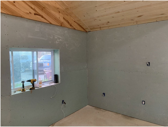
All plumbing, electrical and sewer is instated. Ready to drywall.
