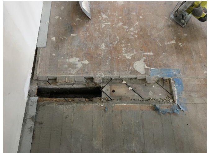
A new floor was installed. First the existing floor needed to be repaired where the wall was removed, then leveled in preparation for new flooring:
