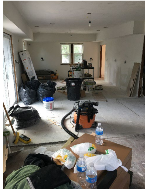
A new floor was installed. First the existing floor needed to be repaired where the wall was removed, then leveled in preparation for new flooring:
