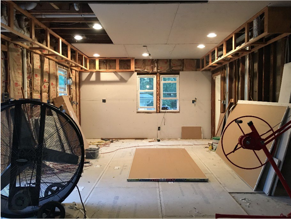
Soffits were added which contain ventilation to outside, plumbing and electrical:
