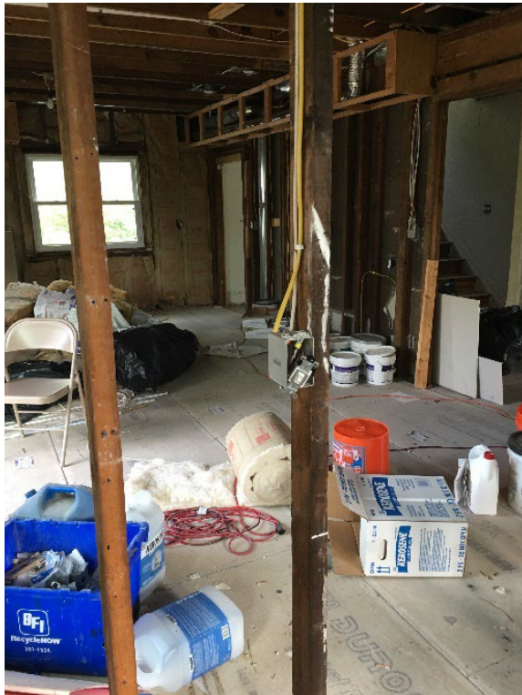
Electric wires and ductwork needed to be removed and reinstalled to accommodate removing the wall to expand the kitchen.
