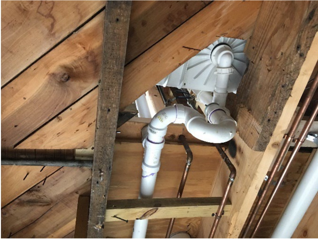
Soffits were added which contain ventilation to outside, plumbing and electrical:
