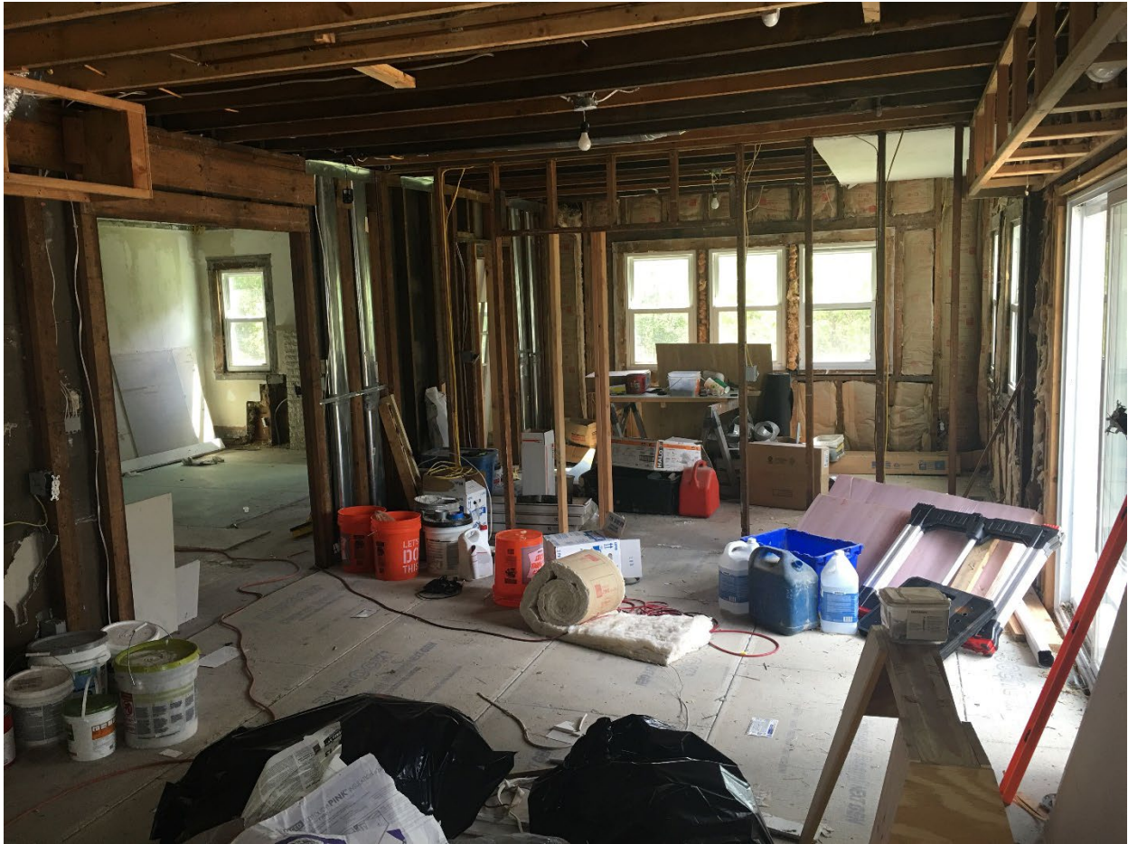
Electric wires and ductwork needed to be removed and reinstalled to accommodate removing the wall to expand the kitchen.
