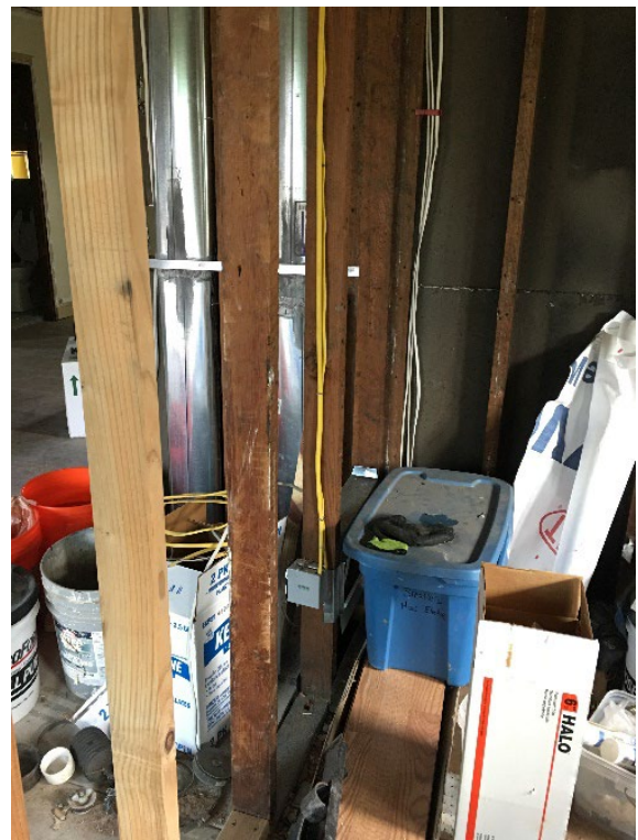
Electric wires and ductwork needed to be removed and reinstalled to accommodate removing the wall to expand the kitchen.
