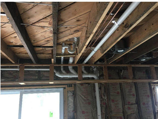
Below are photos of the new plumbing for the second-floor bathroom where a laundry room was added for convenience. There is no longer a need to go down two flights of stairs into the basement to do laundry. The washer and dryer are now on the same floor as the bedrooms.
