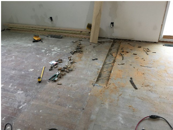
A new floor was installed. First the existing floor needed to be repaired where the wall was removed, then leveled in preparation for new flooring:
