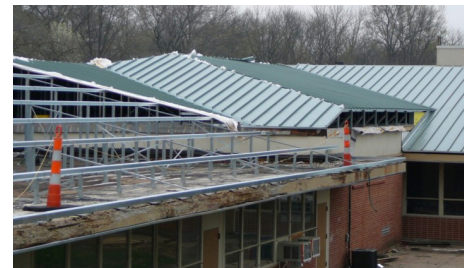
Slope Build-Up over membrane
