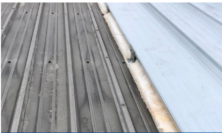
SSR Cover Rib over screwdown roof
