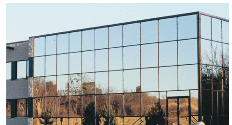
Glass curtain wall with masonry exterior
