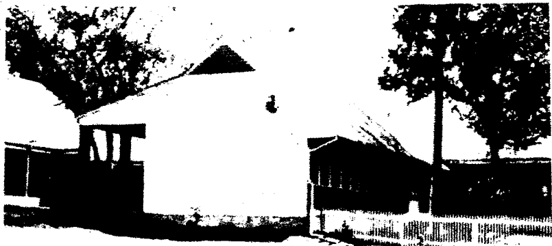
End view of the single-story education wing, constructed in the 1950's
